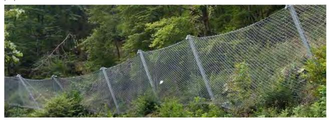
Figure 4 - Example of a rockfall protection fence.
