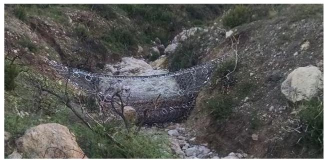
Example of a debris flow fence in a stream channel. The fence works to trap large debris and slow flow velocities.
