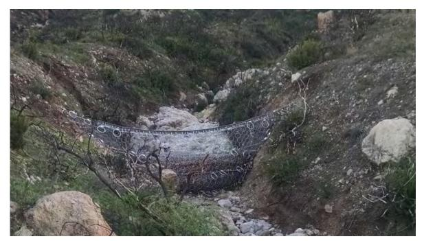
Figure 3 - Example of a debris flow protection fence installed within a stream channel. The fence works to trap large debris and slow flow velocities.
