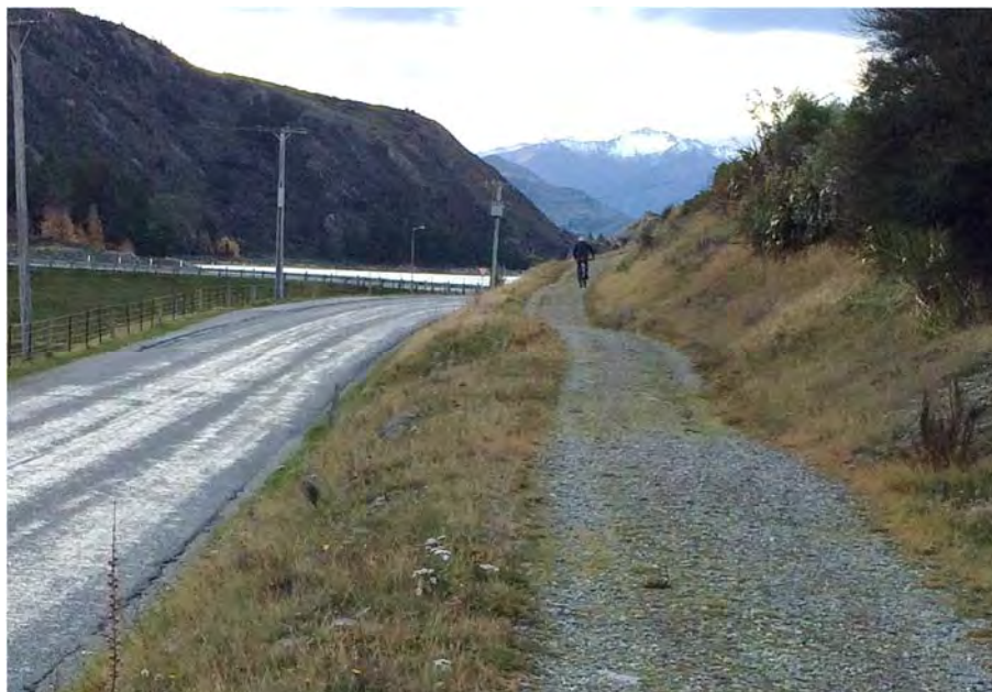
Photograph 7: Elevated Footpath/Cyclepath on Eastern Side of Domain Road
