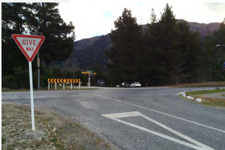
Photograph 2: Cemetery Road / Domain Road Intersection Looking West
