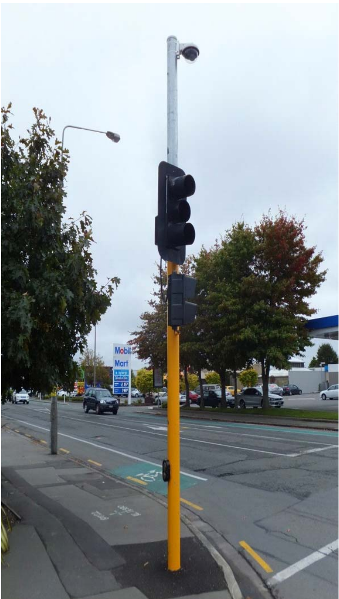
Spunlite Type 2 Combined CCTV / Traffic Signal Pole
