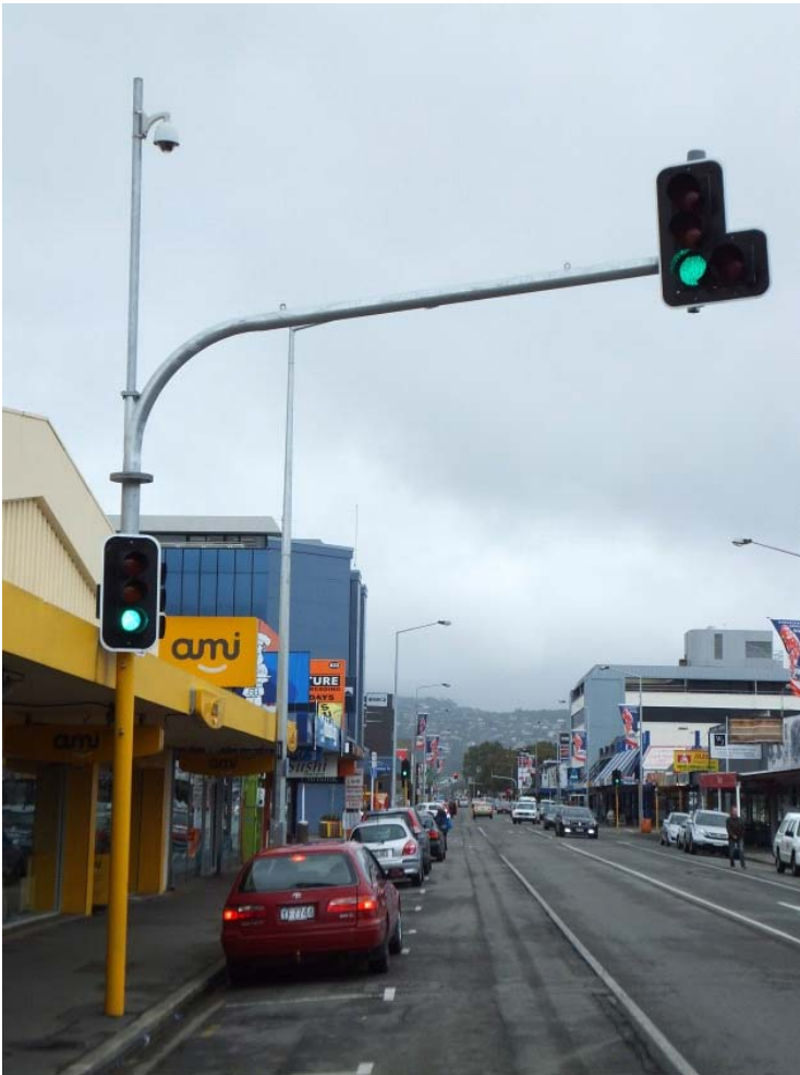
Spunlite Type 5s Mast arm with CCTV / COMMS Extension
