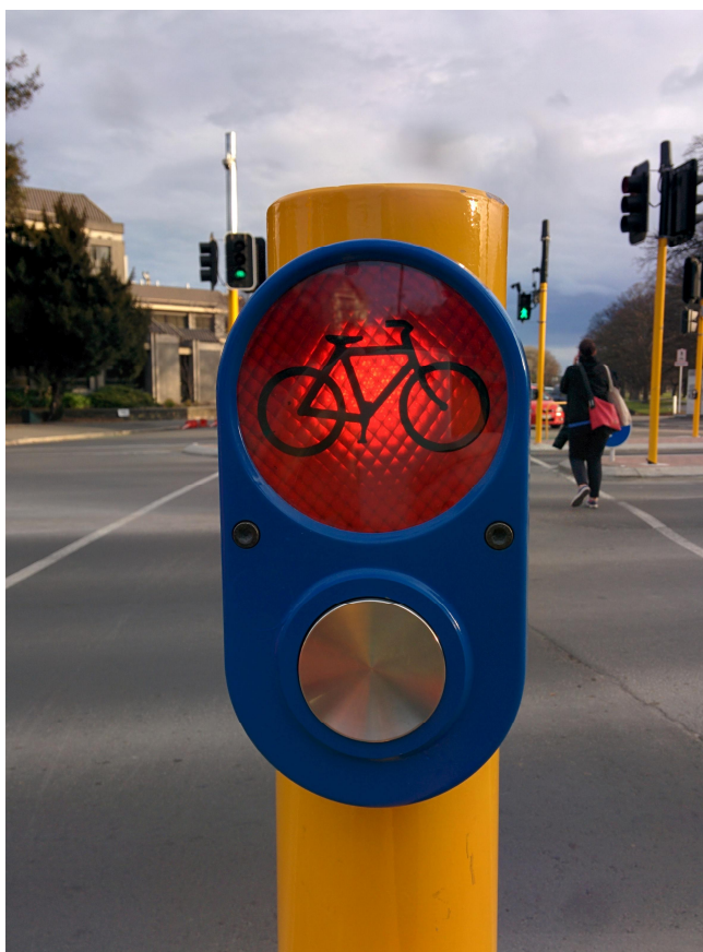
Figure M02 – Cycle call accept indicator displaying call present.
