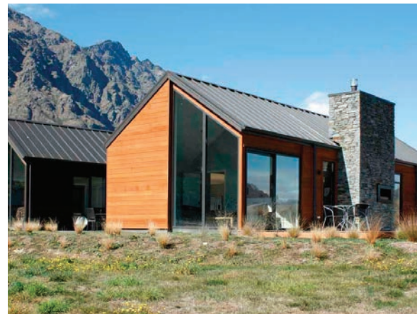
IMAGE 17: ROOF PITCH & MATERIAL
