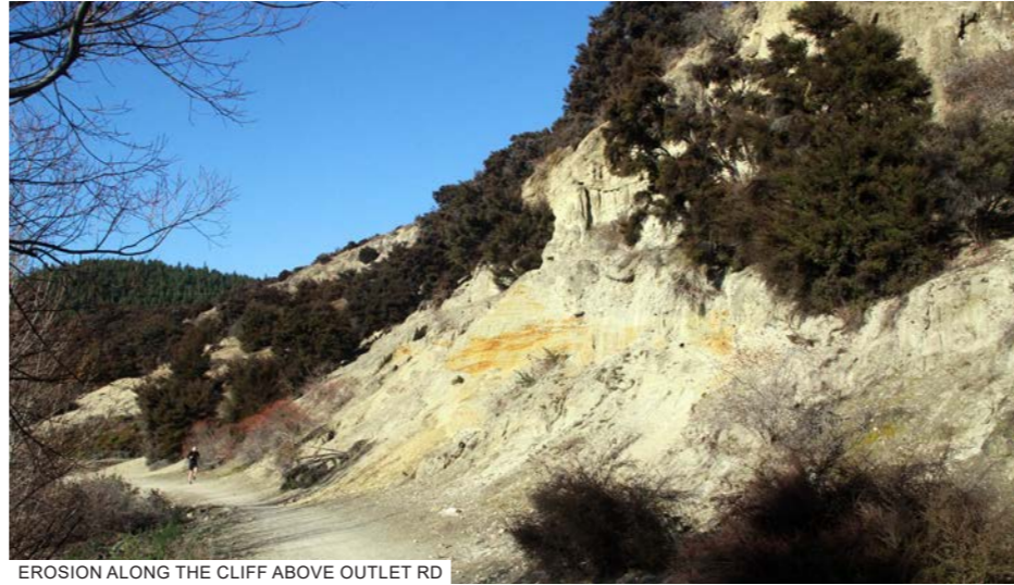
EROSION ALONG THE CLIFF ABOVE OUTLET RD
