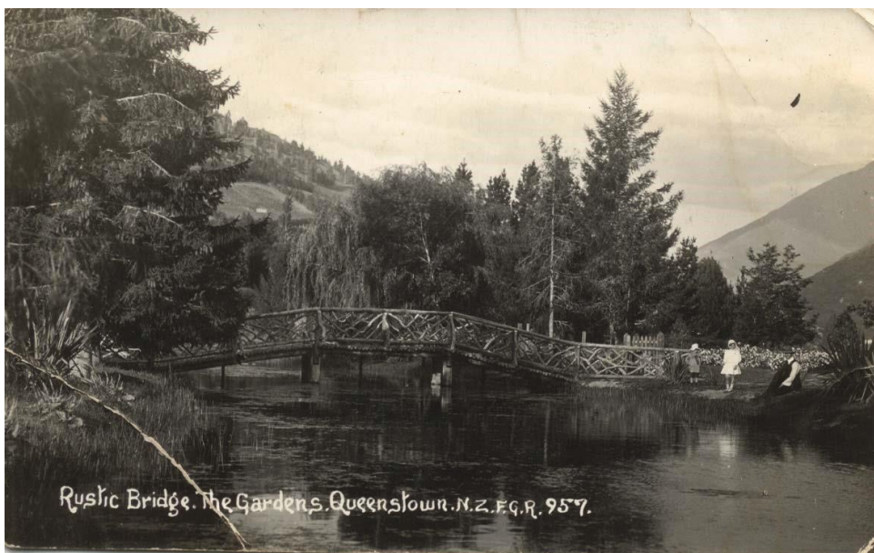
Bridge Queenstown Gardens
