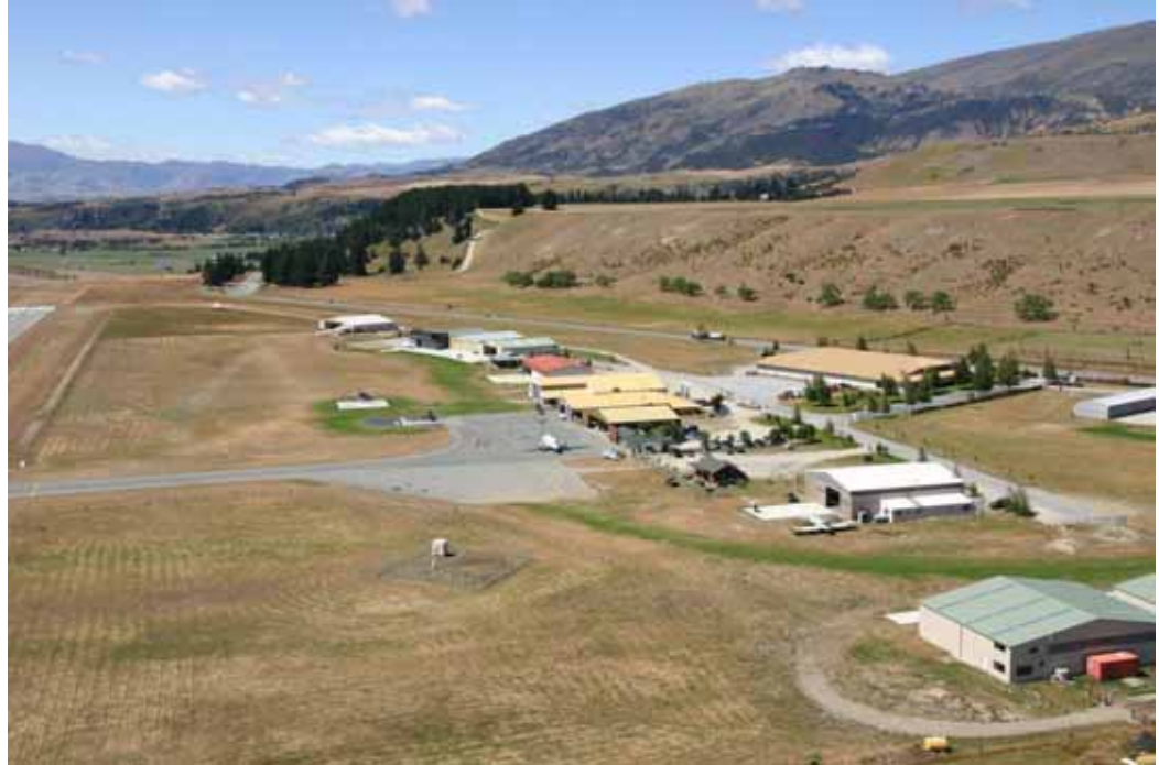
Figure 7-5: This photo shows the existing apron area. The proposed sealed apron extension would extend N out beyond the fuel pumps towards the runway, SE almost to the red roof hangar. The seal would be extended also to the grass section adjacent to the proposed new terminal site
