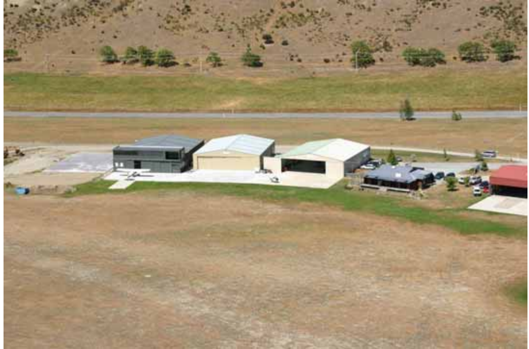
Figure 7-7: Hangars in the Helicopter Zone with existing concrete TALO areas in foreground. The proposed helicopter clearway extends out across the grass to the runway. Note irrigated apron verge to eliminate dust hazard.
