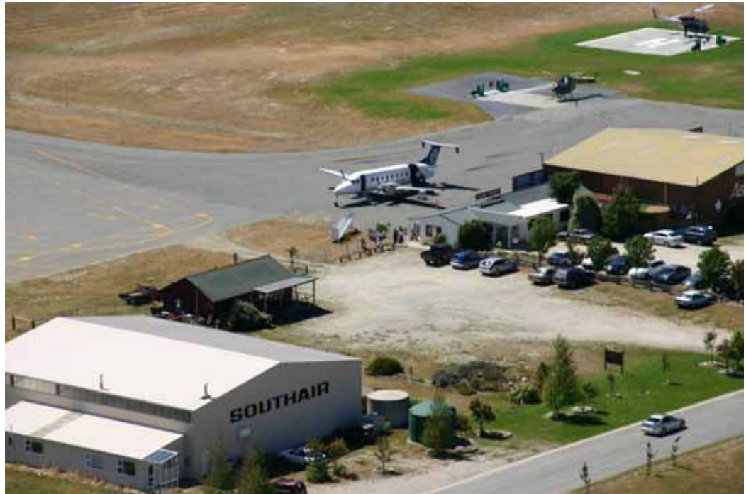
Figure 8-1: Proposed site for new terminal building is located on vacant land between Aspiring Air and Southair including the site occupied currently by the small cottage.
