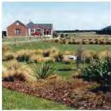
Figure 4.6: Infiltration Basin in a local park along Roydon Drive, Christchurch (Source: Waterways, Wetlands and Drainage Guide, CCC, 2003)
