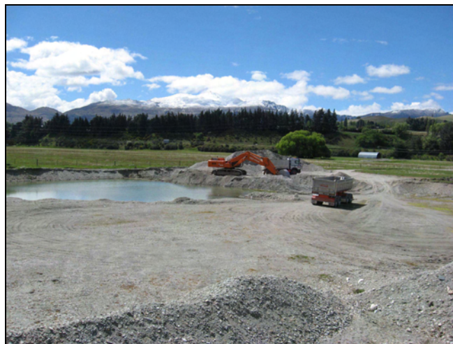
Photo 1: Height of Ground Water Table is Apparent from this Gravel Extraction Pit on the Lower Terrace
