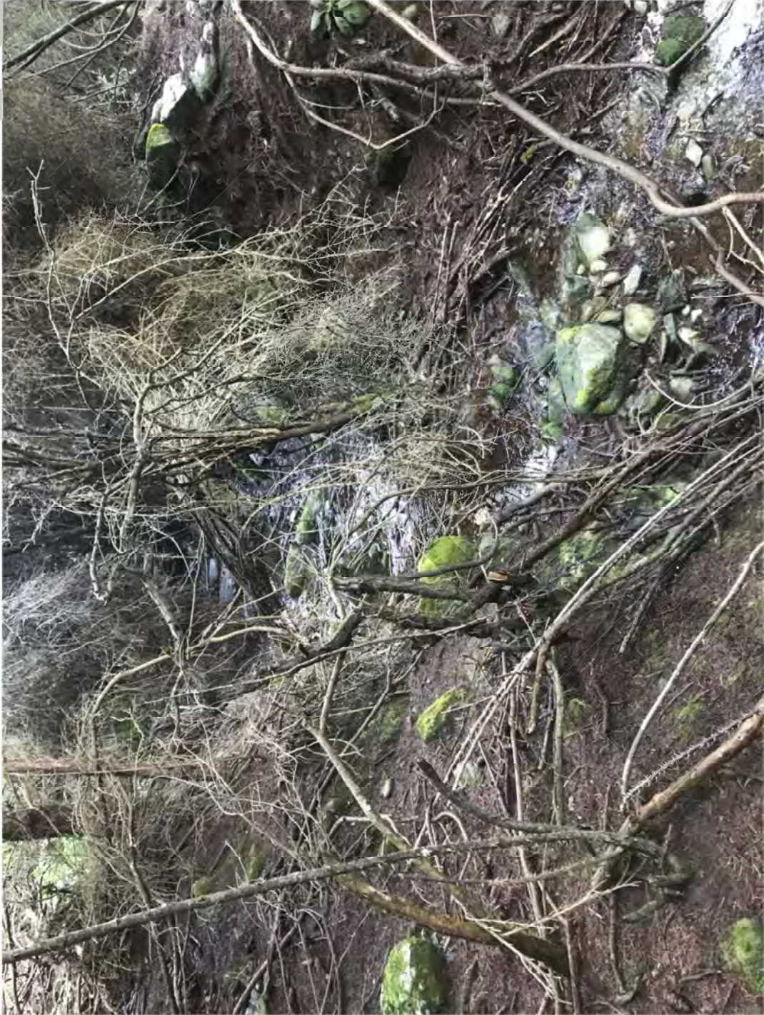
Photograph 4: Middle Creek channel. RL ~430 above the site. Showing limited coarse material from debris flood deposition in the depositional zone.
