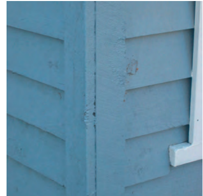
Painted Weatherboard with boxed corner.
