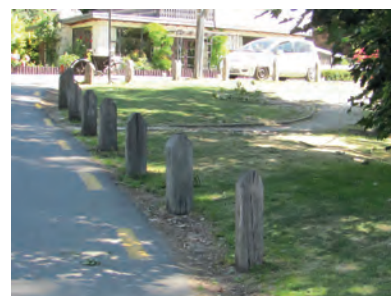
Good example of simple timber bollard.
