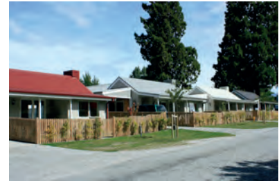
New development on Suffolk Street located within LDRZ reflecting scale, layout, fencing and simple planting reflective of the adjoining ARHMZ.
