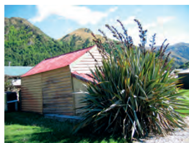
Sheds or outbuildings are highly characteristic accompaniments to Arrowtown Cottages.
