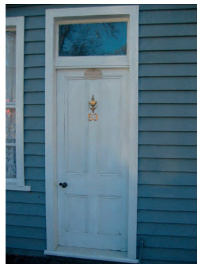
Frame and panel door with top light.
