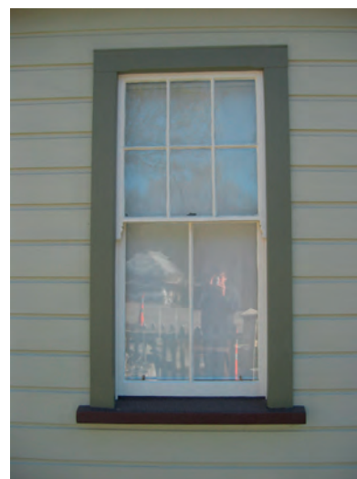
Window -double hung with lattice.
