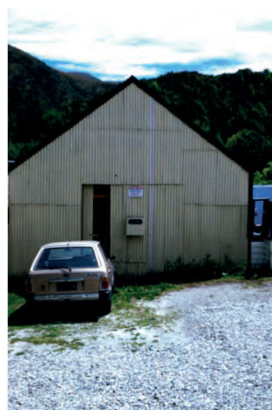
The simple back of a false front shop primary element as seen from the Lane.
