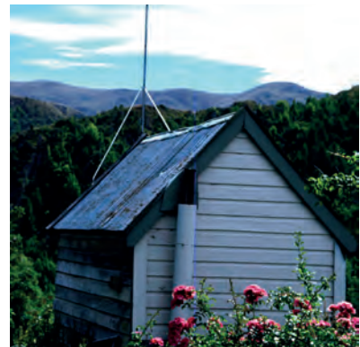
Small shed-out building.
