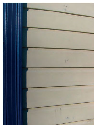
Timber weatherboard.
