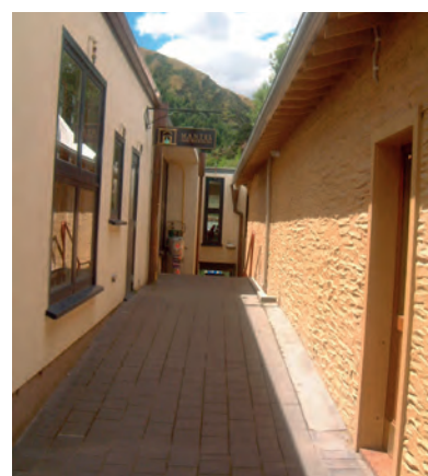
Uninteresting pedestrian link with poor detailing.
