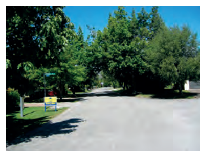
Thompson Street has characteristics of the old town eg narrow carriageway, no kerb & channel, grass verges & trees.
