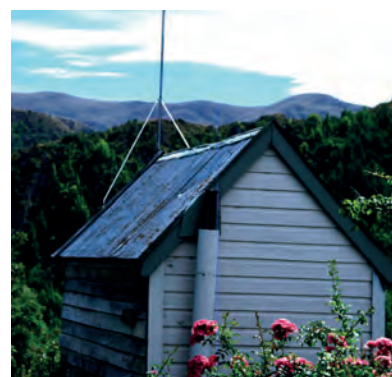
Shed, 18 Wiltshire Street.
