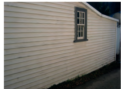
Painted Weatherboard with boxed corner.
