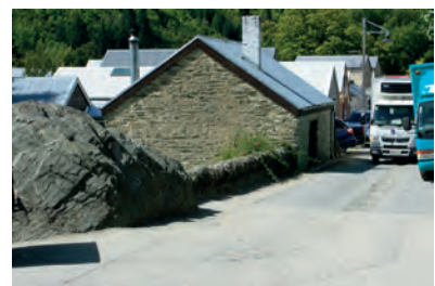
Looking north along Arrow Lane, showing the relationship between lane and buildings, with buildings typically erected hard up against lot boundaries.
