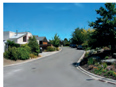
Do not plant or place stones or boulders on the verges.
