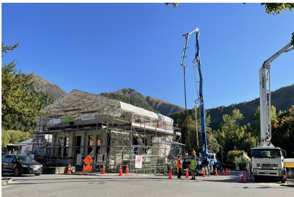
Seismic strengthening work underway, 24th March 2021.
