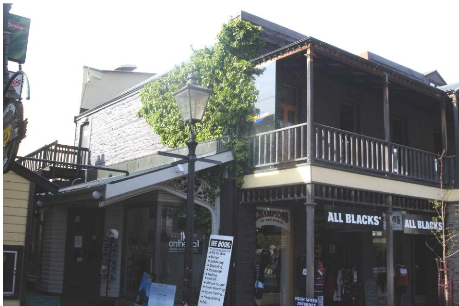
The Queenstown Athenaeum and Town Hall, 17 Ballarat Street
