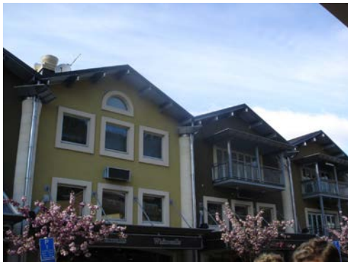
Stratton House, 24 Beach Street
