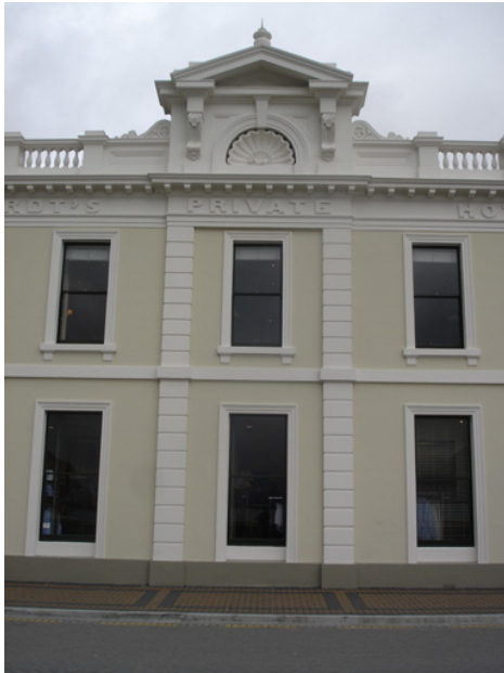
Eichardt's Hotel (painted plaster)
