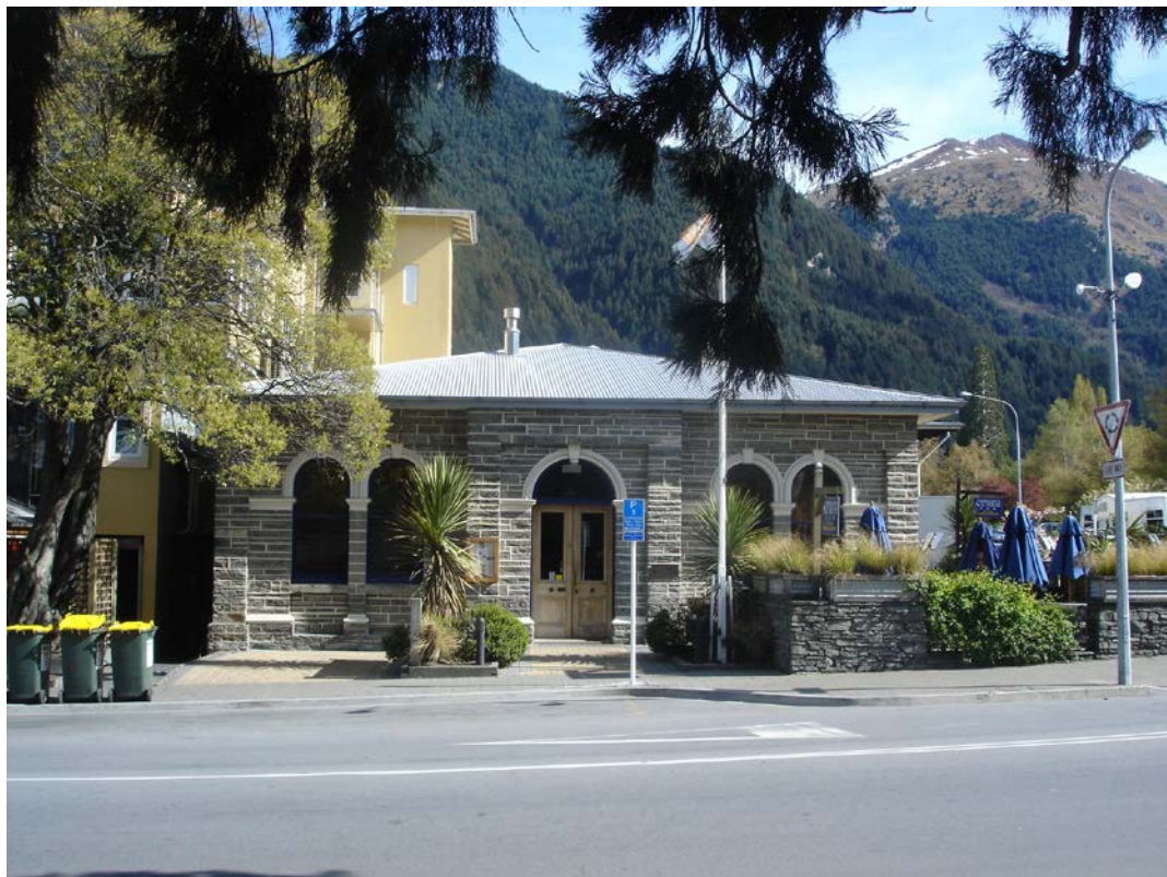
Old Council Chambers, Ballarat Street.
