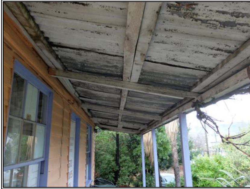
Figure 12 The veranda roof structure.
