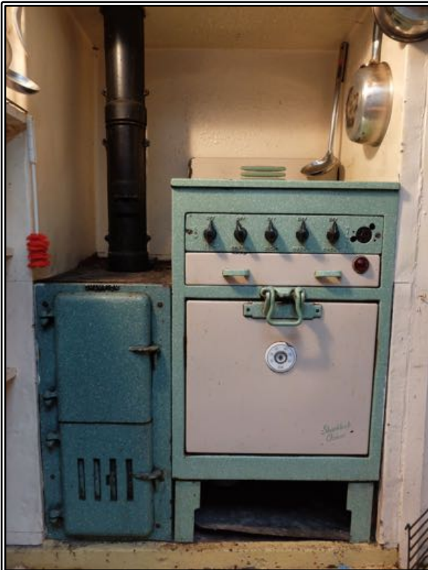
Figure 28 The Champion destructor on the left and Shacklock Orion electric stove on the right. Both are in typical 1930s green (& cream in the case of the cooker) enamelled colour schemes.
