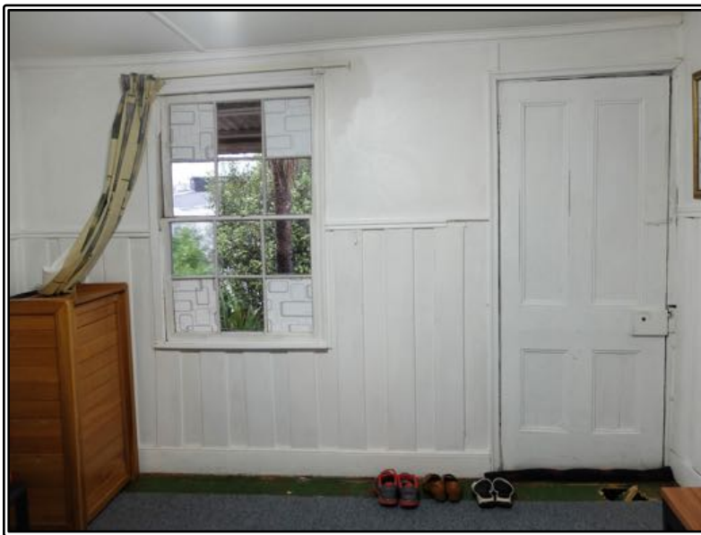
Figure 19 The front wall of the living room, showing the door, window and wainscot.
