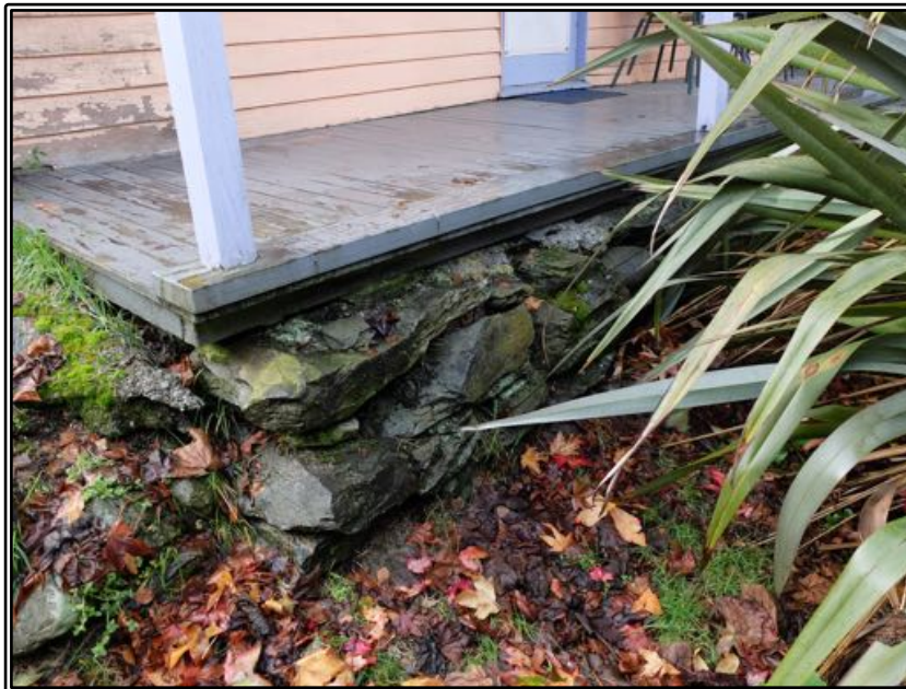
Figure 13 The veranda deck and supporting stone revetment.
