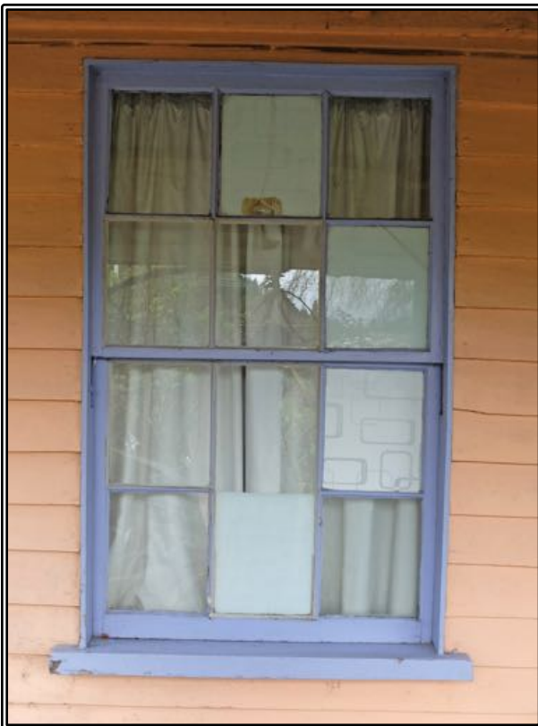
Figure 11 The left hand (north) front sash window of the cottage.
