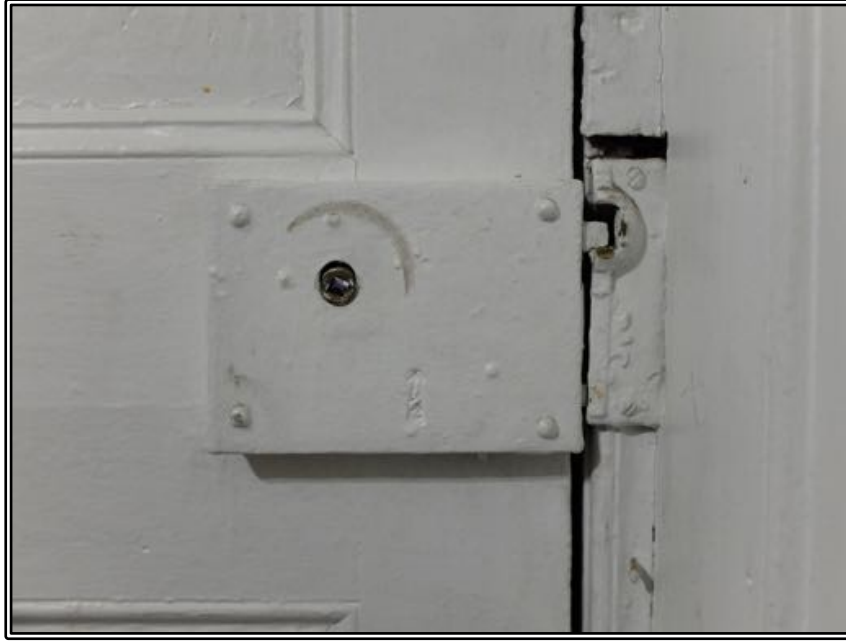
Figure 23 The front door lock, with the doorknob removed.
