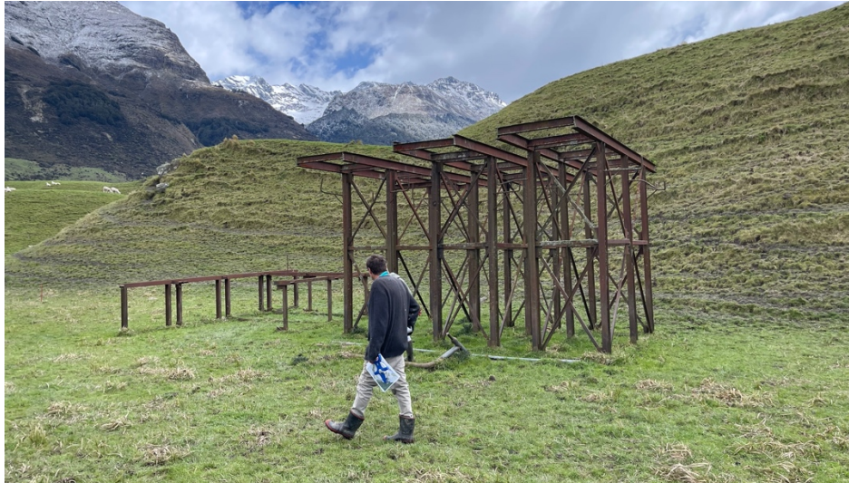
Figure 9. View of construction supports
