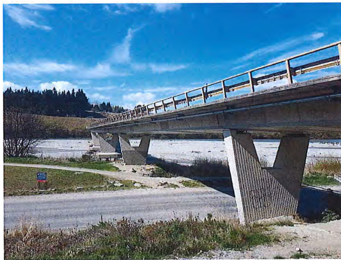
Figure 1 – Shotover River Bridge
