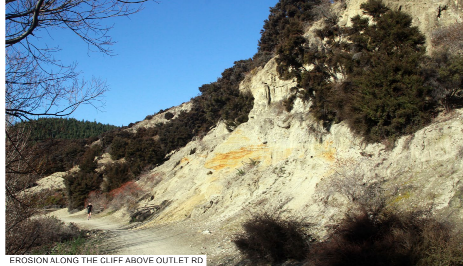
EROSION ALONG THE CLIFF ABOVE OUTLET RD
