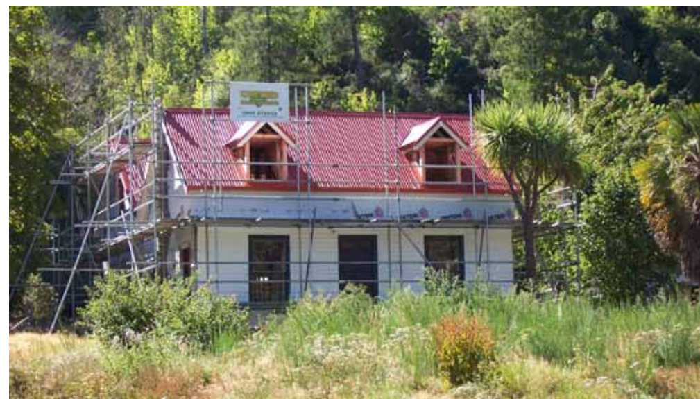
Closeburn Homestead restoration Recipient of Heritage Incentive Grant
