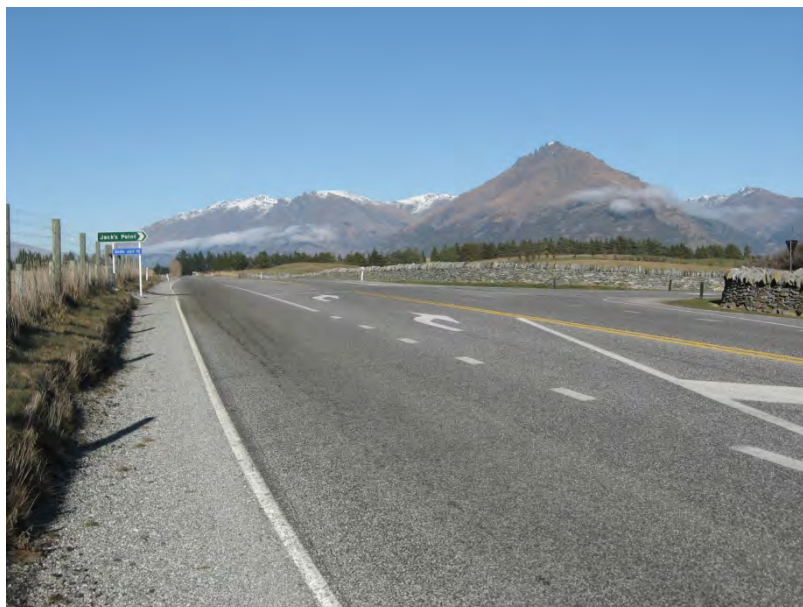
Photograph 3: SH6 looking south towards Maori Jack Road intersection
