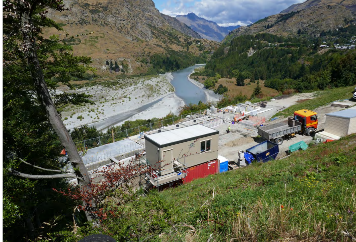
Photograph 8: View over Onsen Pools extension to Shotover River (photograph taken at 50mm lens equivalent on 22-02-19)
