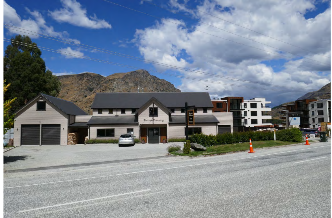
Photograph 9: Commercial development within the zone (photograph taken at 50mm lens equivalent on 22-02-19)
