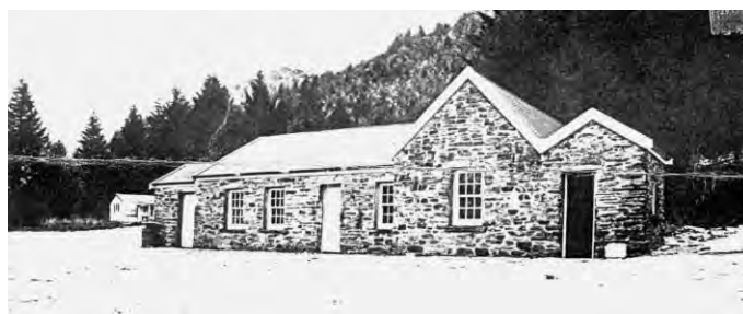
Restored Skippers school 1992 (LDM, N 886)
