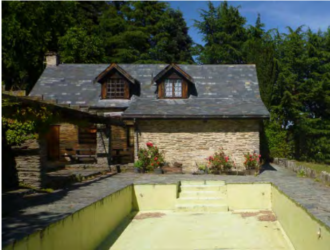
Condition of The Loose Box as of December 2013
