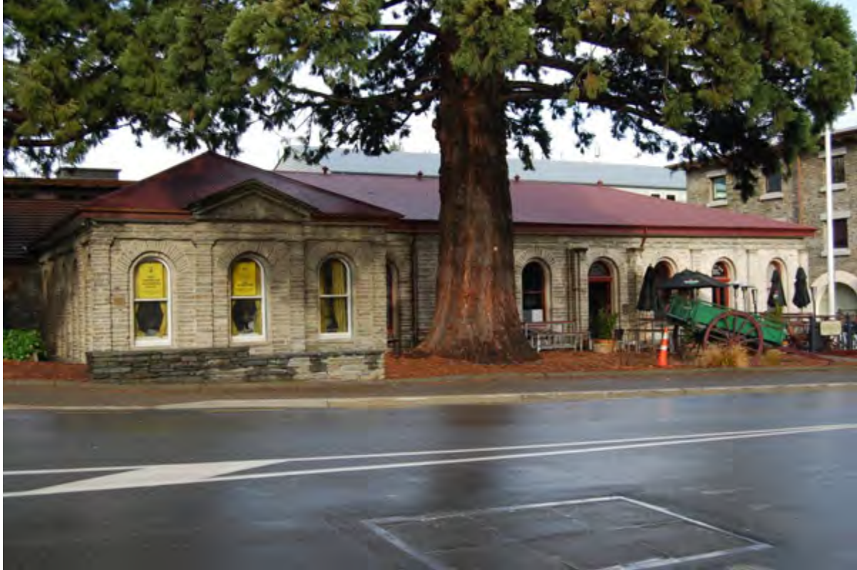
Queenstown Courthouse, November 2013.
