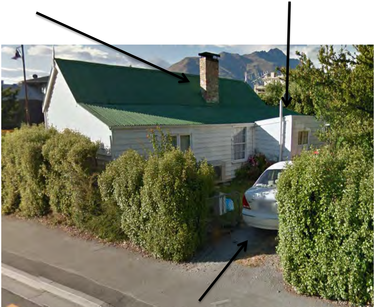
Image Three: Note the added annex, chimney and added driveway.
