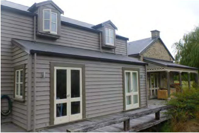
The additions to Douglasvale and the original stone building.
