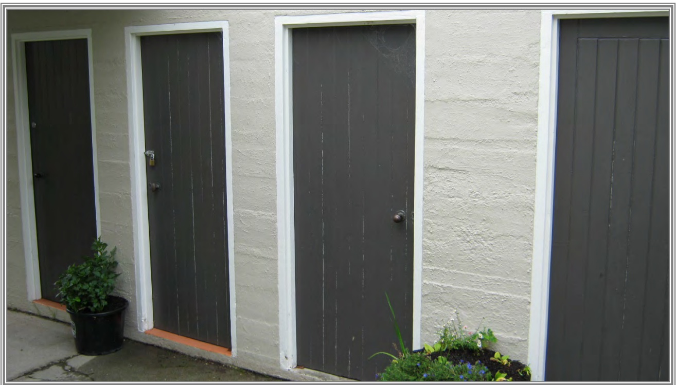
Fig. 2, Showing the outbuildings to the rear of the homestead.
