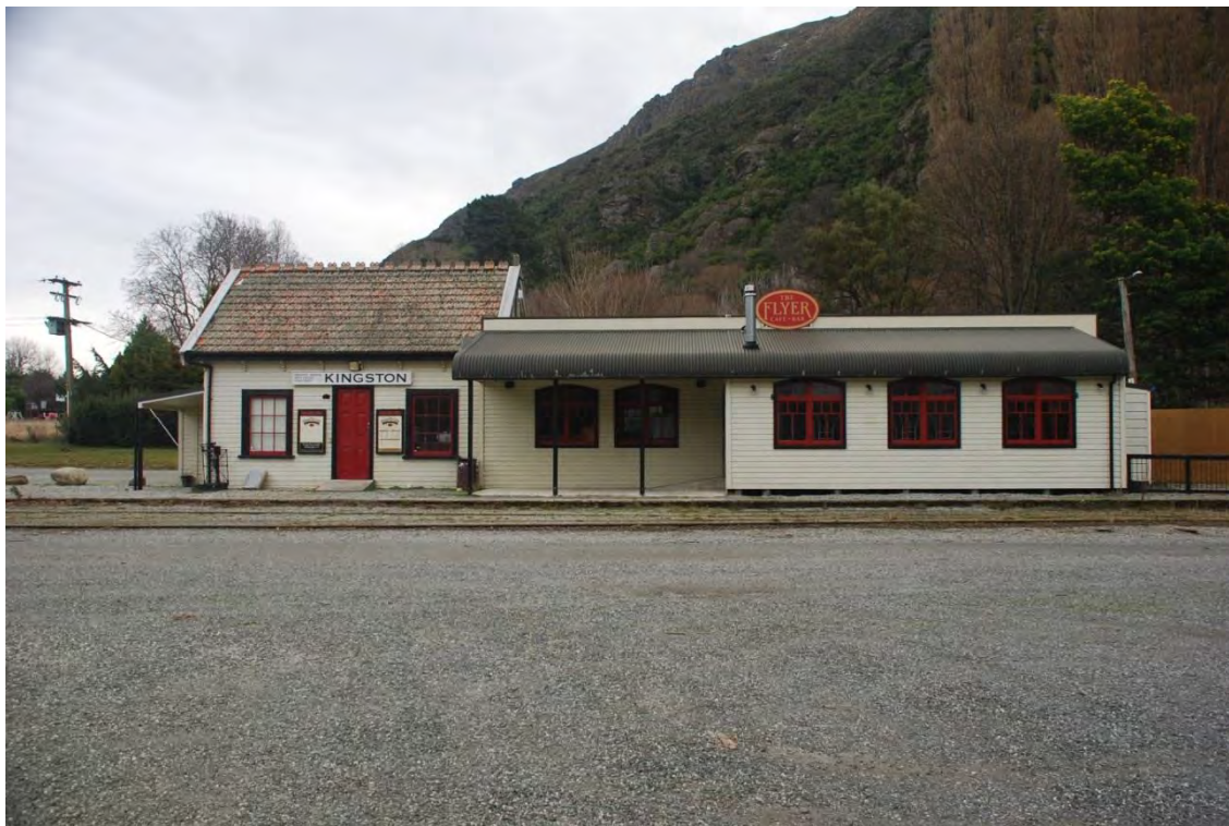
Photo 11 The 1973 Kingston Station building is on the left of the photograph and has the Marseille tile roof. The building adjoining on the right is a later addition.
