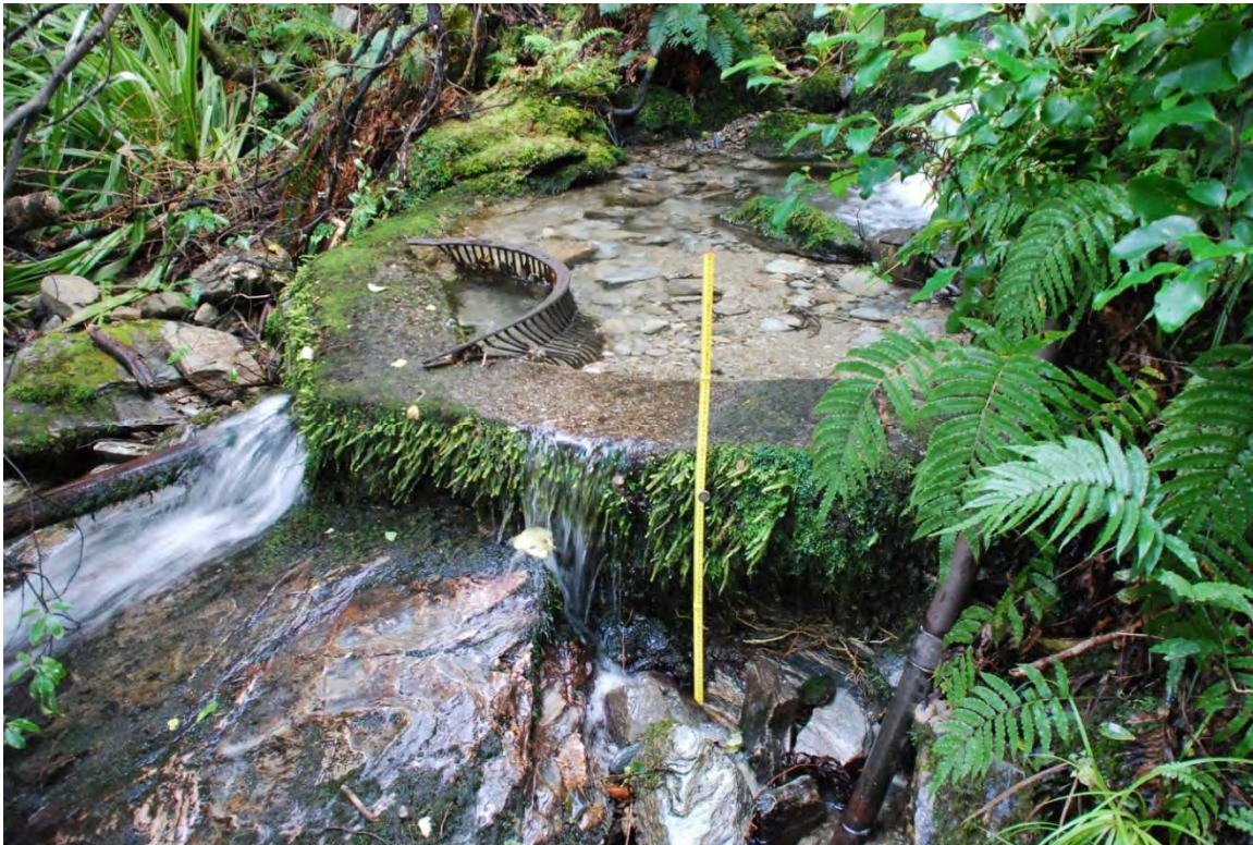
Photo 1 Concrete weir and iron grill (with yellow 1000mm rule for scale)
