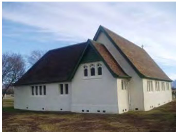
Rear of church
