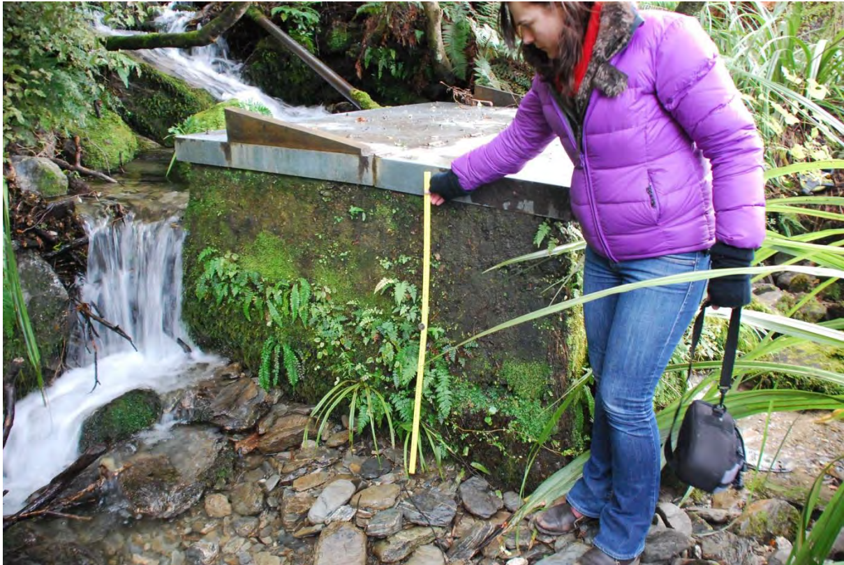
Photo 4 The concrete storage tank with (modern) galvanised steel lid.
