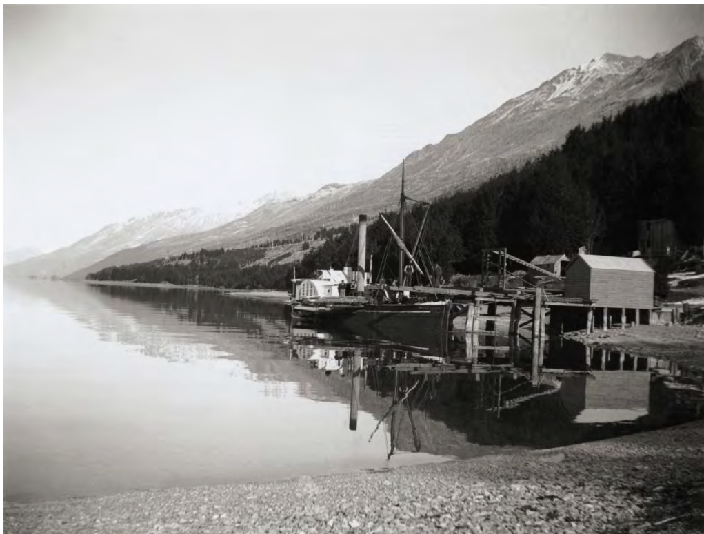
An un-dated photograph of the Antrim pile-driving at the jetty with the wharf building clearly visible. Single rows of piles can be seen followed by two rows of double piles where the jetty has been extended out into the bay. The shape of the jetty closest to the ship has also changed (S13-090e Hocken Collections Claude Burgess coll. neg. P00-025-080).
