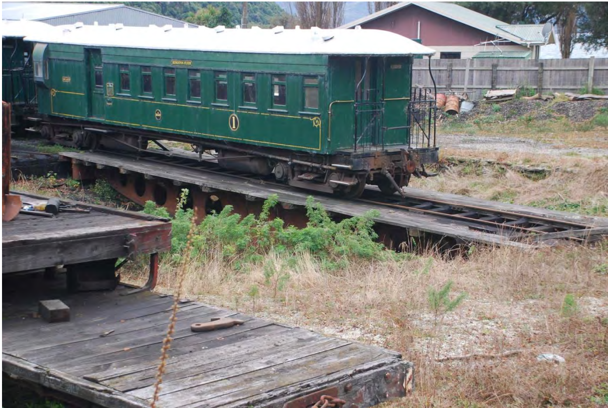
Photo 1 The turntable with circular perimeter wall of stone in the Kingston station yard/depot
