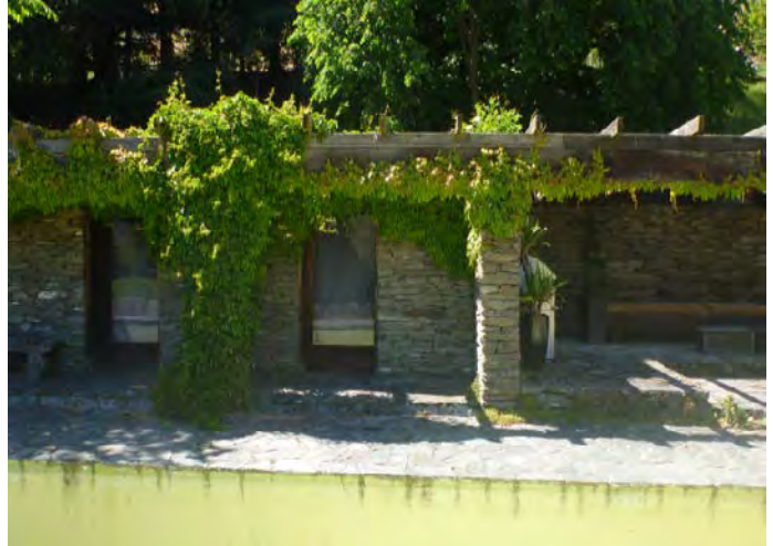
West facing wall of new extension, December 2013
