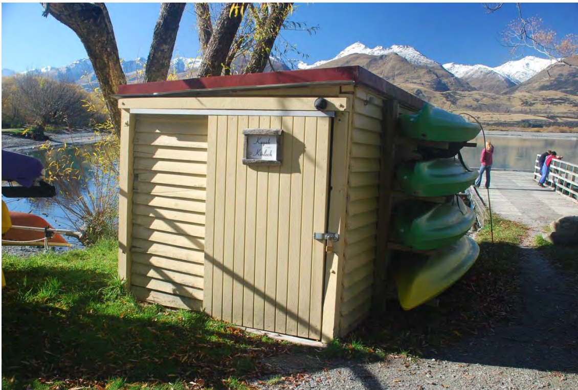
The wharf building with former opening blocked-up where the kayaks are and a new opening/sliding door in the west elevation.
