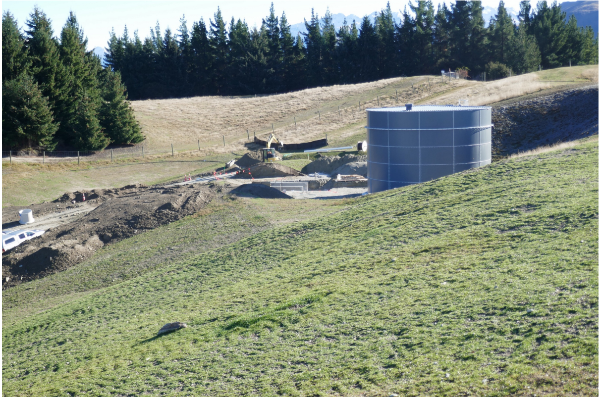
Photograph 1: existing water tank approved under RM200889 (photograph taken at 50mm lens equivalent on 24 May 2022)
