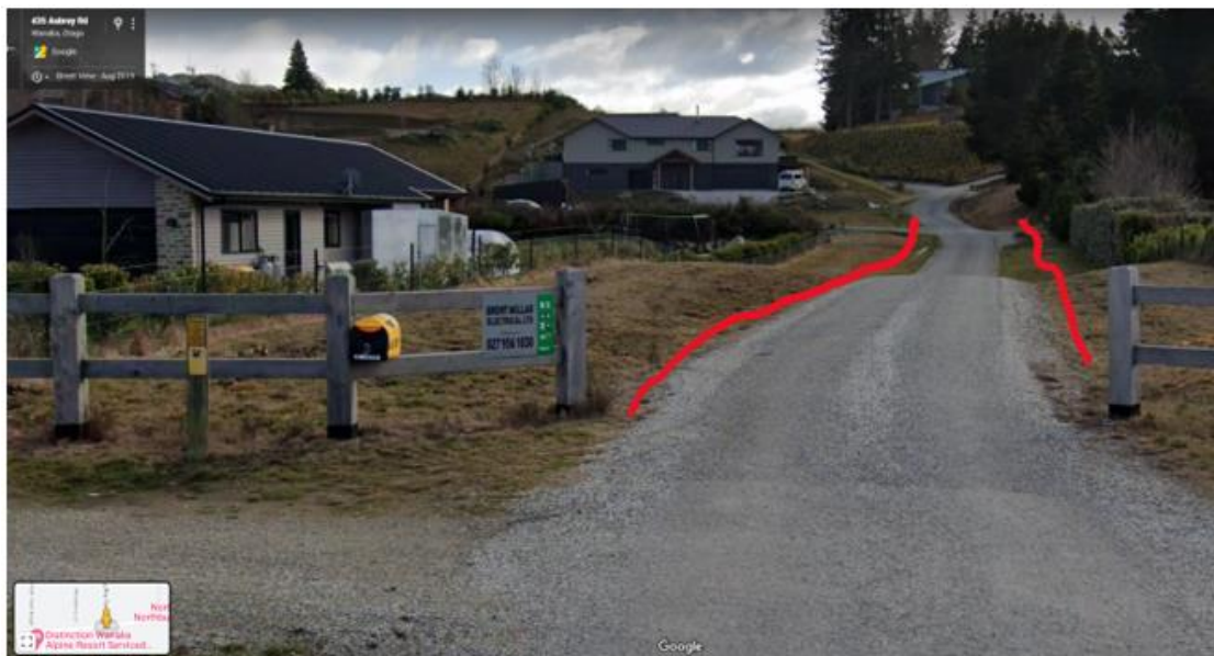
Figure 10-4 Bottom of the Mt Roy Terrace with its "bunds" visible on each side. The soakage pits are located on each side of the road depression between two houses
