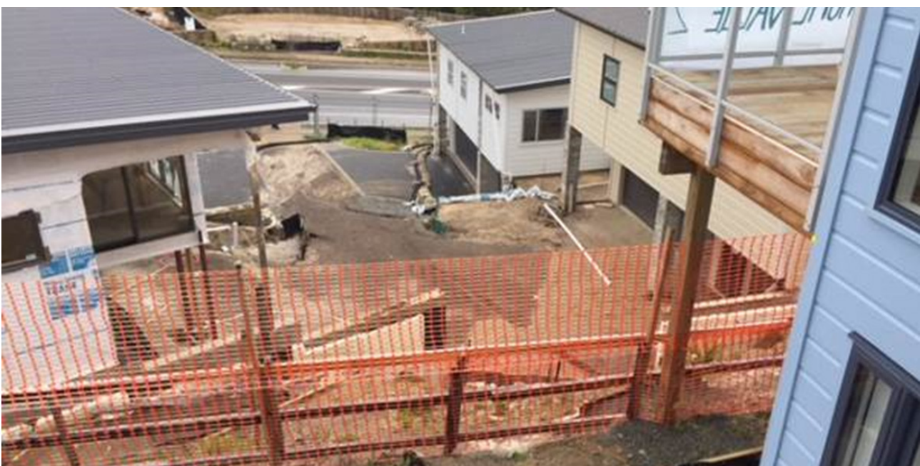
Figure 3: View from 5 Aneta Way over houses at 307, 307A, 309, 309A Lakes Boulevard
