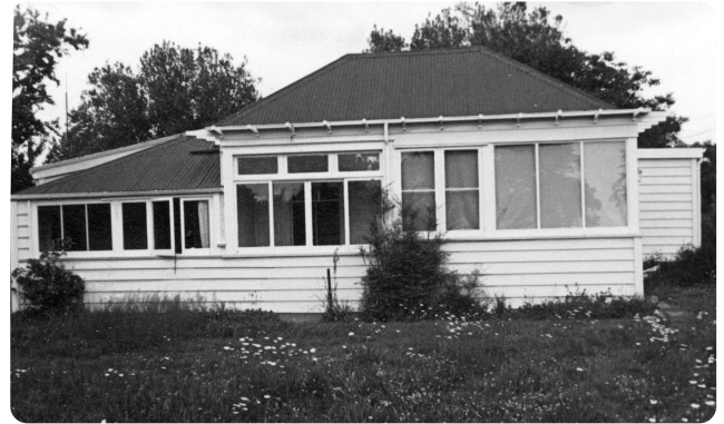
Figure 12 - World first New Zealand all electric home.
