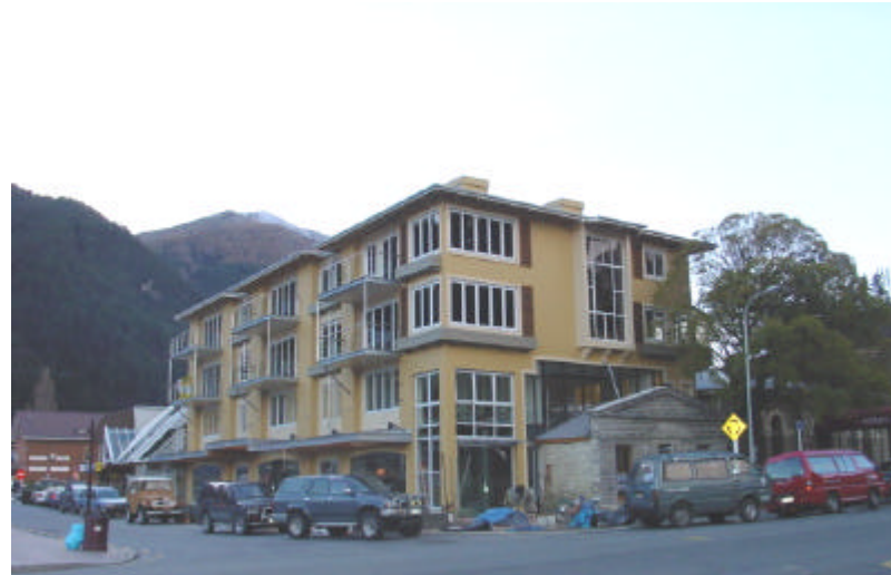
Box 39: Mixed use in the Queenstown CBD - retail at the street frontage, apartments above
