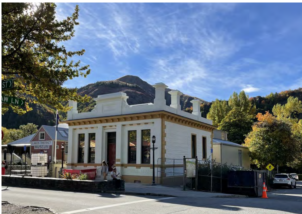
The 1875 BNZ Building restoration nearing completion in April 2022
