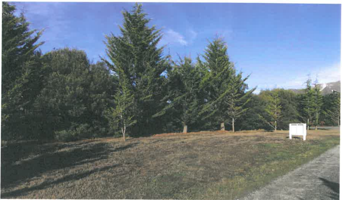
Cypress and Eucalyptus planting screening substation on south boundary of site.
