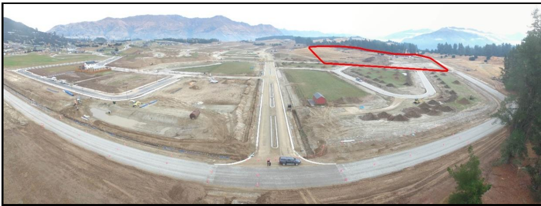
Figure 1: Drone photograph westwards over Outlet Road 2017 showing ongoing construction March 2017
