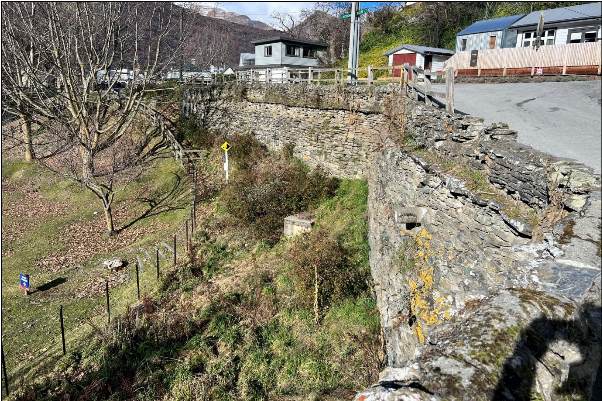
Figure 2. Butler's Green wall looking east along Buckingham Street.
