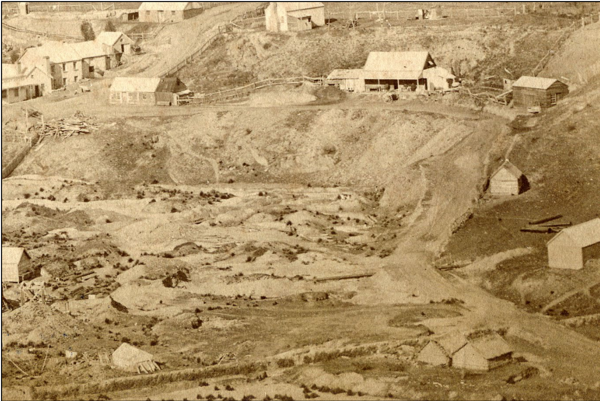
Figure 3. The unretained bank of Buckingham Street from the township to the Arrow River and Bush Creek, circa 1874. 5
