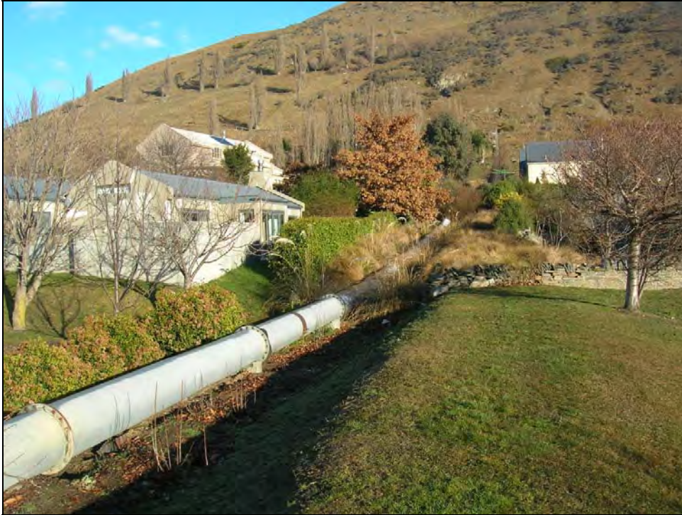
Figure 6: Arrow Irrigation infrastructure passes through the residential development
