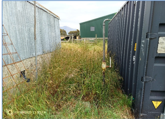
Photo 2: Possible underground fuel tank at the northern edge of the shed.
