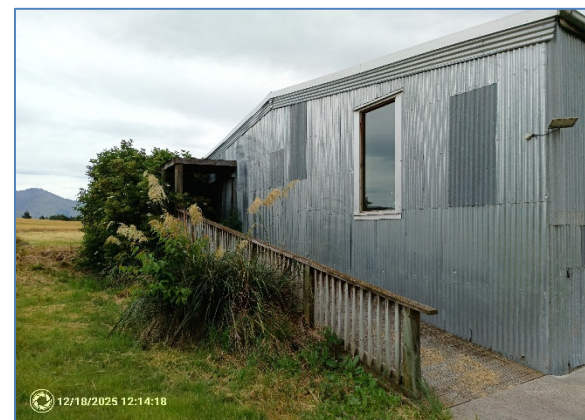
Photo 9: Walkway on the southern side of the shearing shed.
