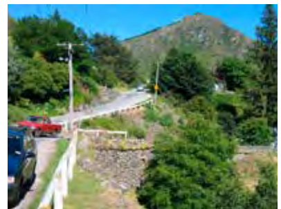
Butlers wall, Villiers Street behind.
