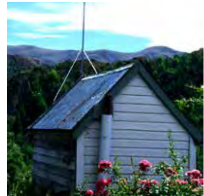
Small shed-out building.
