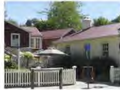
New development to the rear of the Postmaster Restaurant, viewed from eastern end of Buckingham Street, reflects contemporary two storey development incorporating simple shed forms in a grouped arrangement of buildings.
