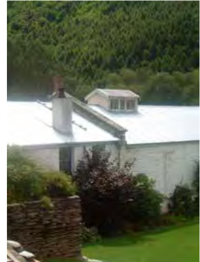
Side walls predominately solid.
