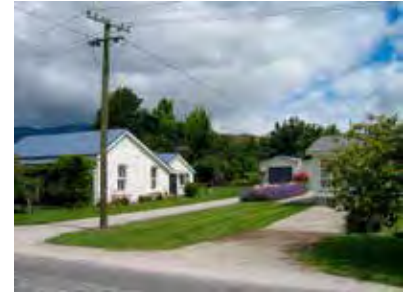
Garage set to rear of section.
