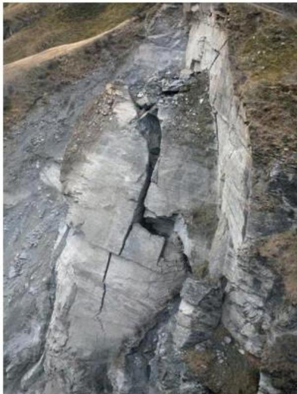
Figure 9. Photo of the 2008 slip before it was released by water jacking
