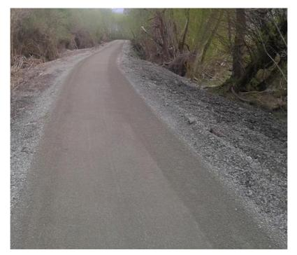
1.6.10. To achieve optimum compaction, water shall be sprayed onto the aggregate surface. Compaction will be deemed complete when a well bound pavement surface is achieved which is free of voids and loose stone.
