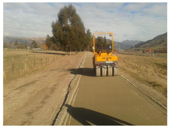
1.6.6. A 5-10mm layer of crusher dust shall be used to cap the aggregate layer and provide a smooth riding surface.
