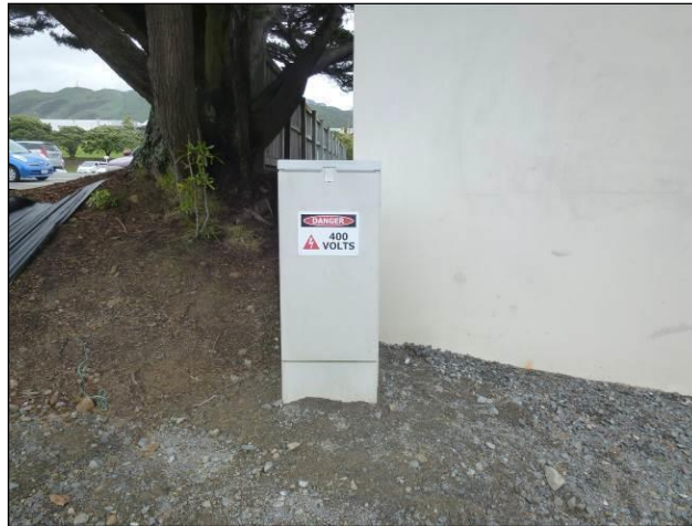
Figure 2: Typical Distribution Pillar
