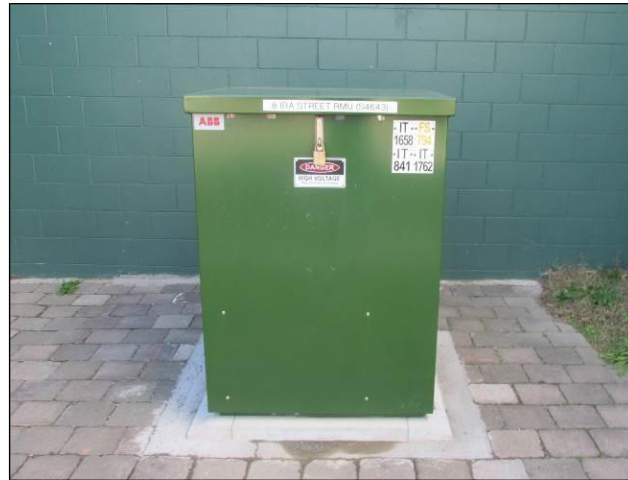
Figure 3: Typical 11kV Ring Main Unit
