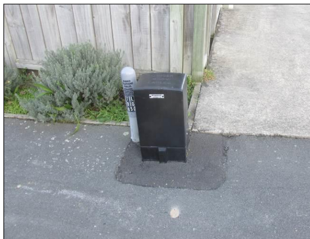
Figure 1: Typical Service Fuse Box
