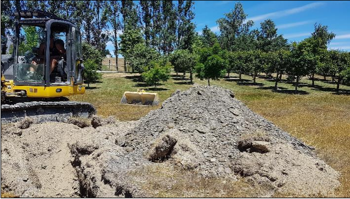
Photo 1: Looking south across Lot 2, indicates the gravel material excavated from Test Pit 2.
