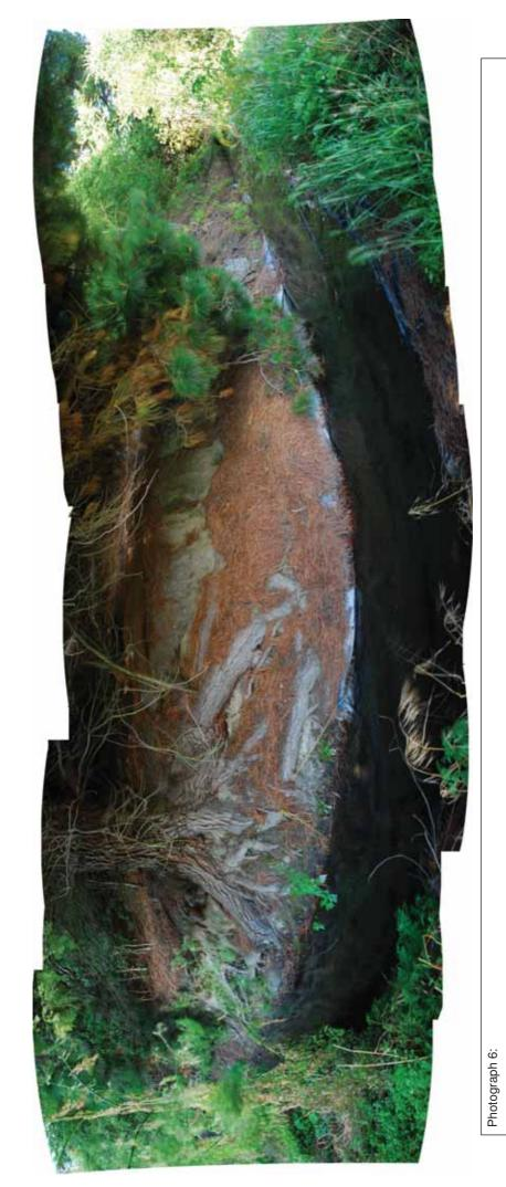
Part of the Arrow Irrigation race as it runs along the slope of the hillside. The race is still very much in use and ongoing maintenance is clear to see along much of this stretch. The black plastic lining to the race has been put in recently, going by the relatively unweathered appearance of the plastic, probably within the last 5 to 10 years.
