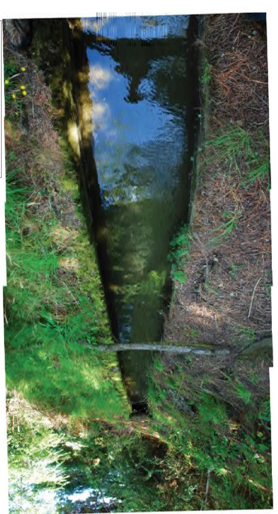
The culvert probably dates to the 19020s/30s, as there is no indication that the concrete has needed repair or patching up.
