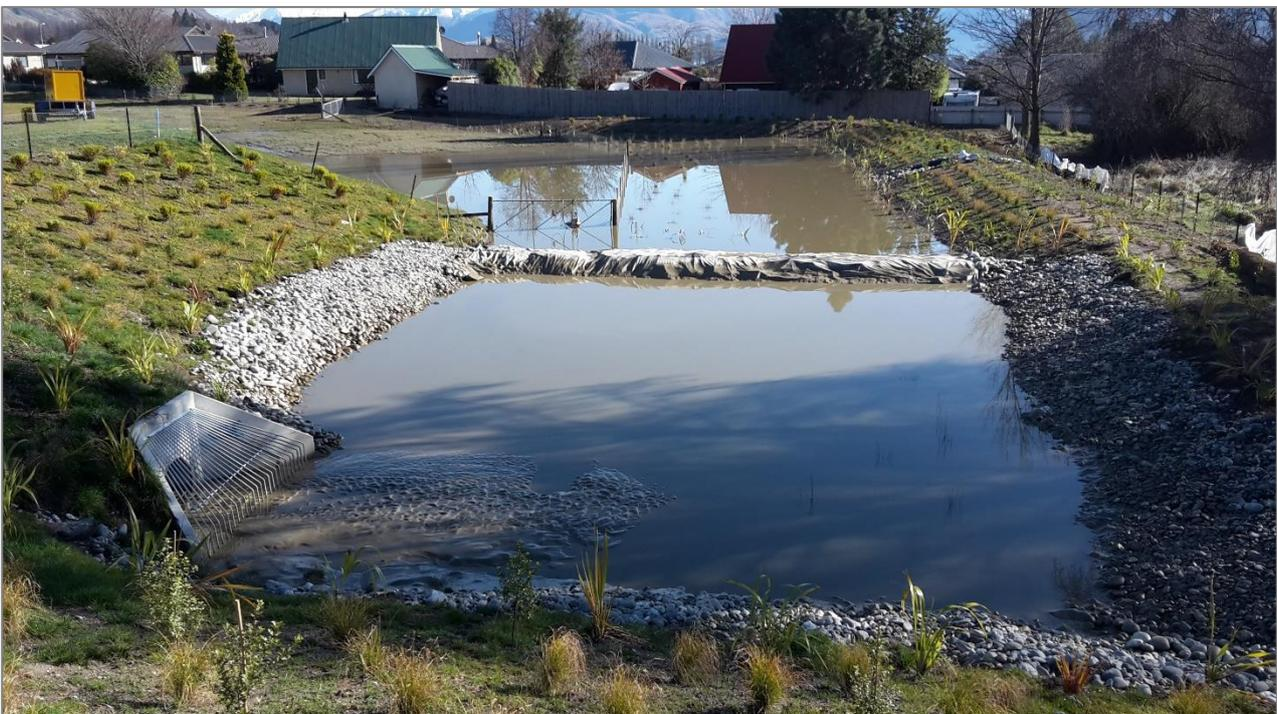
Figure 7: Sediment collected in a completed stormwater pond from Figure 6 catchment (the stormwater pipe was half full of sediment and will require extensive mucking out)
