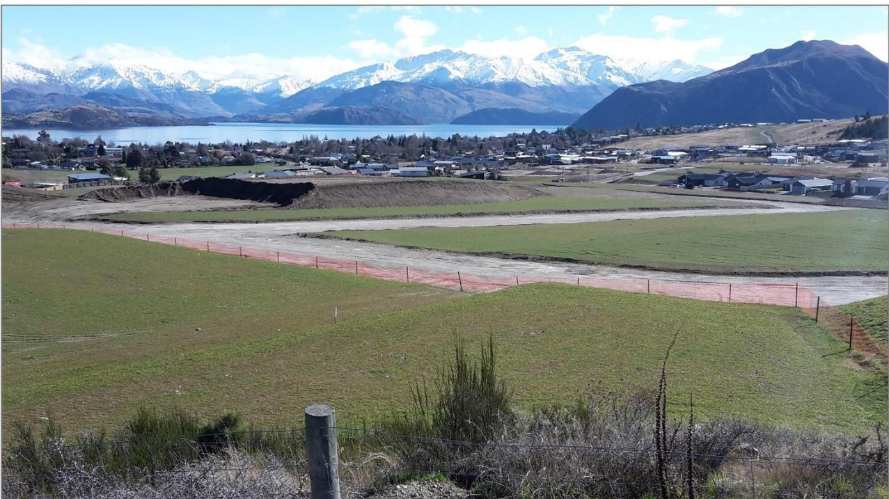
Figure 5: Unstabilised topsoil stockpile
