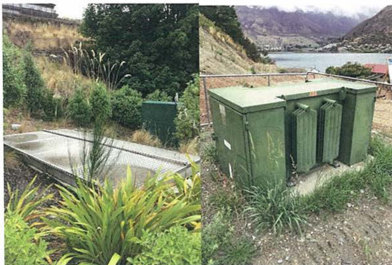
Photographs 1 & 2. Middleton Road Pump Station & Transformer. Source – Patterson Pitts Group
