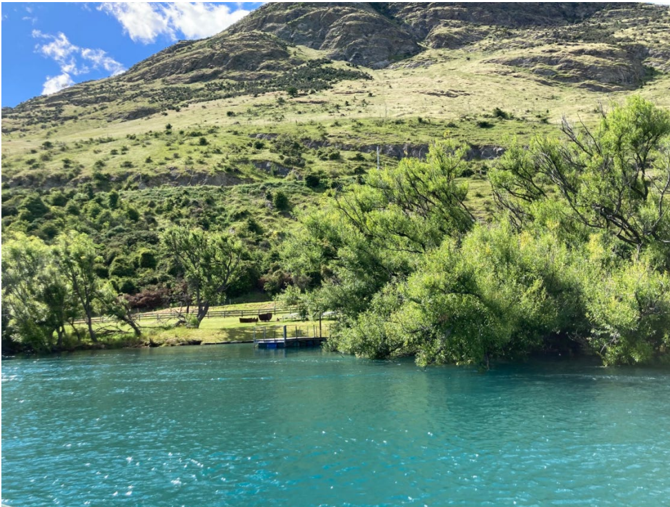
Figure 9: View of jetty from river when passing directly past location (between screening vegetation).
