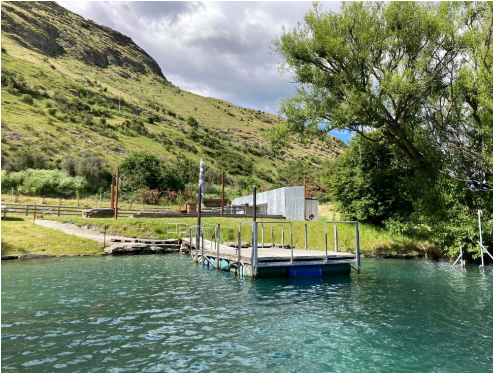
Figure 2: Confluence Jetty (looking west)
