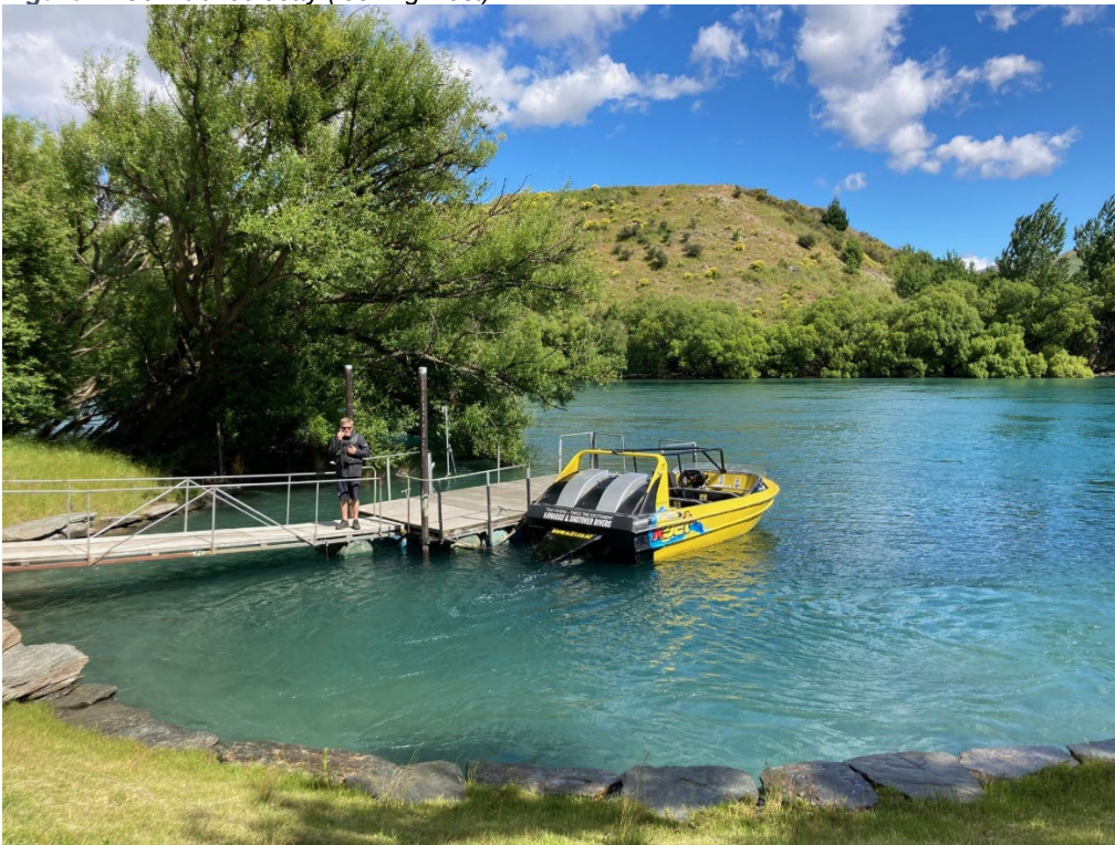
Figure 3: Confluence Jetty (looking east)
