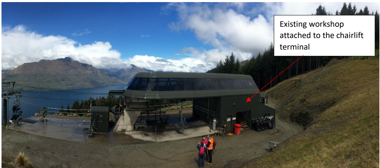
Figure 2: Photo of the existing chairlift top terminal and workshop
