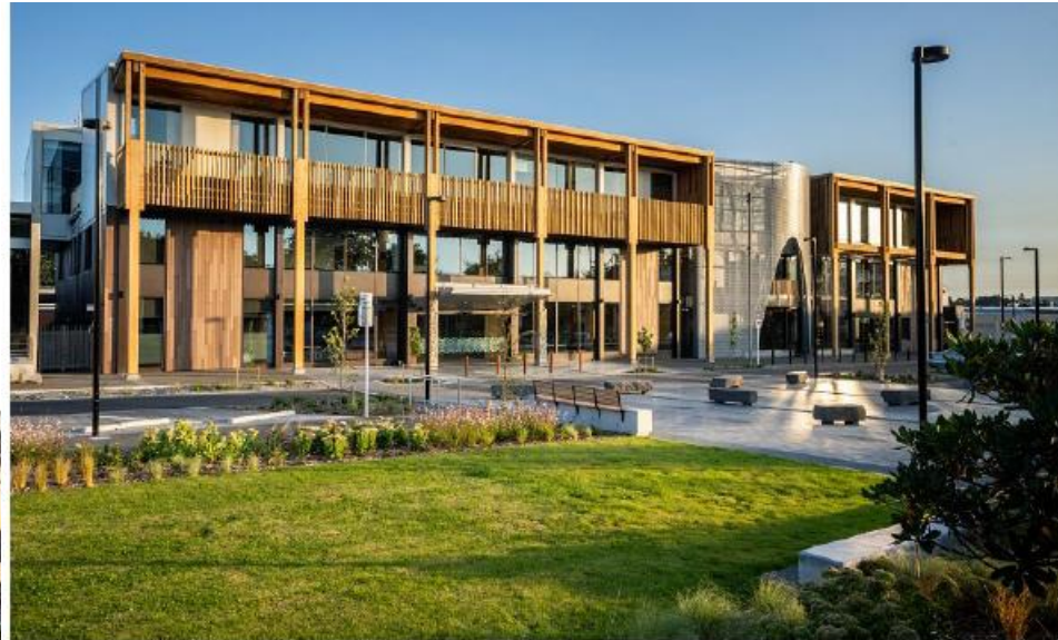
Figure 4: Ashburton Library & Civic Centre | Te Whare Whakare – Existing Adapted and Purpose-Built CAB
