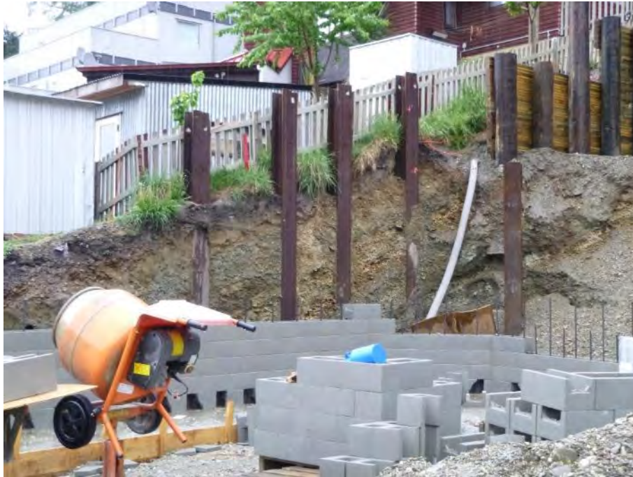
Figure E 2 - Alluvial fan and beach deposits at 62 Fryer Street (under development, 2018).
