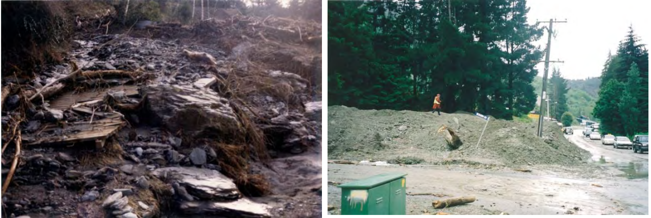
Figure 4 - Debris from the May 1986 debris flow on Brewery Creek Fan (left); and the 1999 event at the intersection of Bowen Street and Gorge Road (right). After ORC, 2011.
