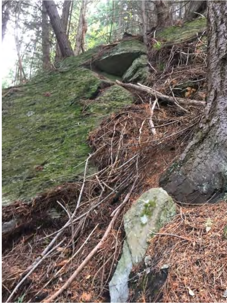
Figure E 32 - Photograph taken from base of cliff looking upslope and showing block fallen from cliff onto slope blow (45.114299; 168.392974; 540m asl).
