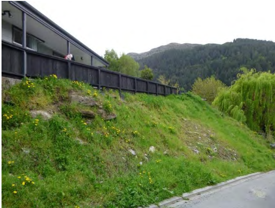
Figure E 1 - Alluvial fan deposits in the upper fan adjacent to 45 Boydtown Way, with boulders visible (2018).
