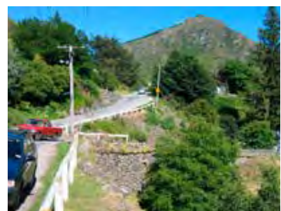
Butlers wall, Villiers Street behind.
