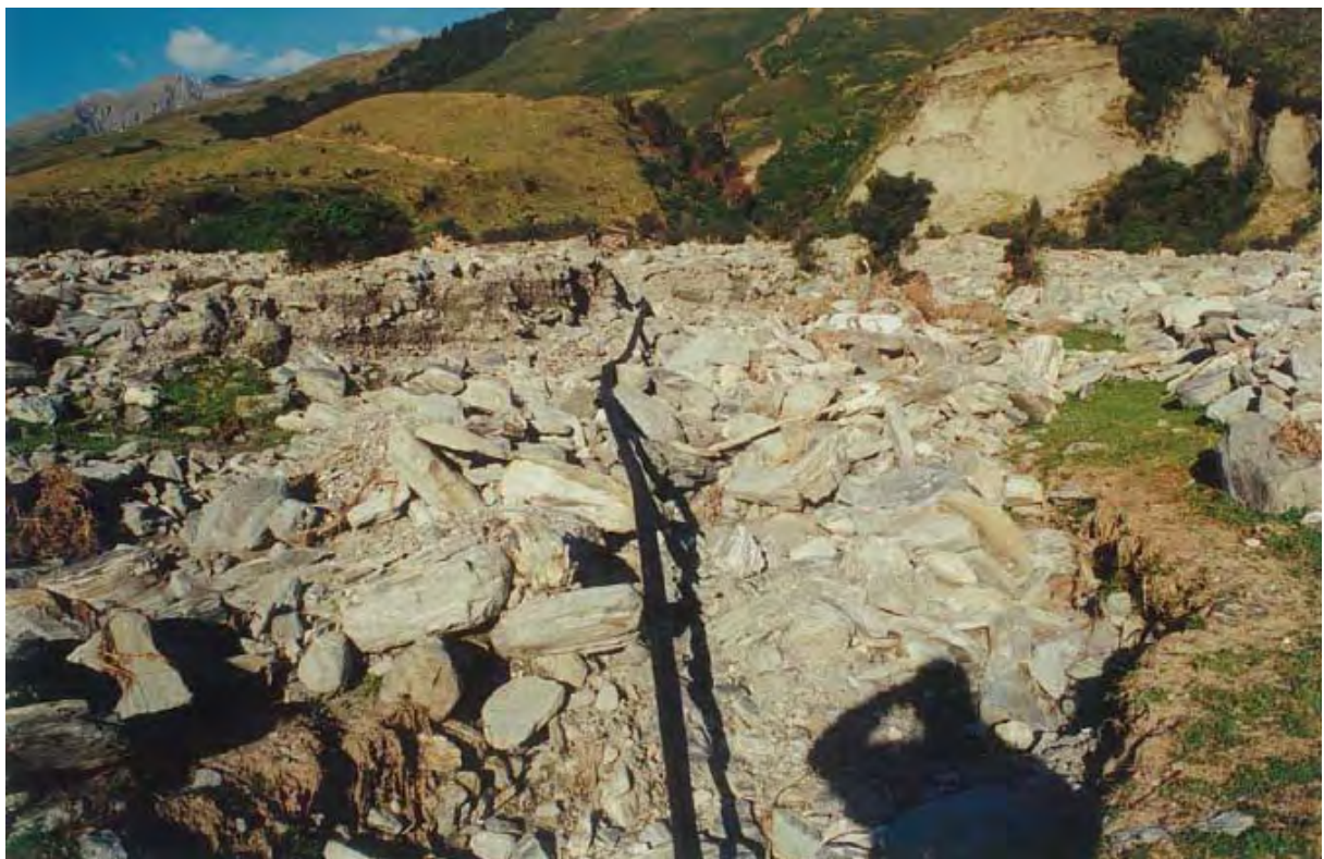
Figure 24: Water pipeline to intake, Ewings Creek (1994).
