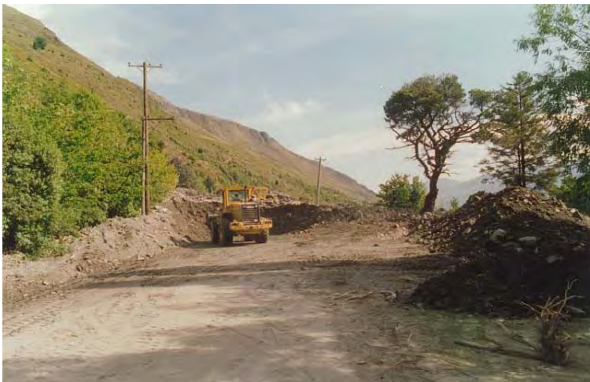
Figure 13: Clearing SH6, Wharf Creek, 1994.
