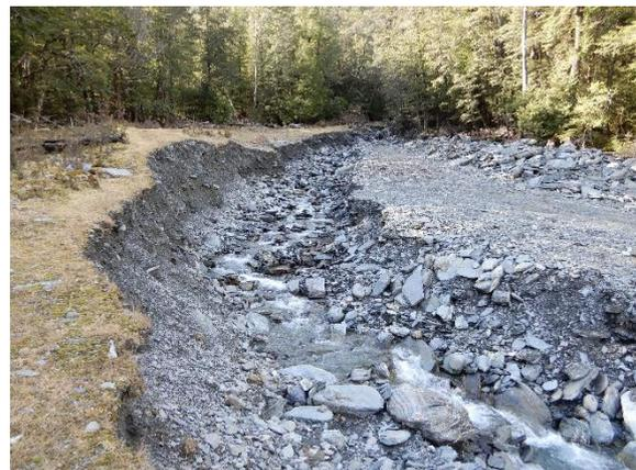
*Photo 7: Cassells Stream in upper reaches of fan where several levee breaches have occurred prior to channel clearance.*
