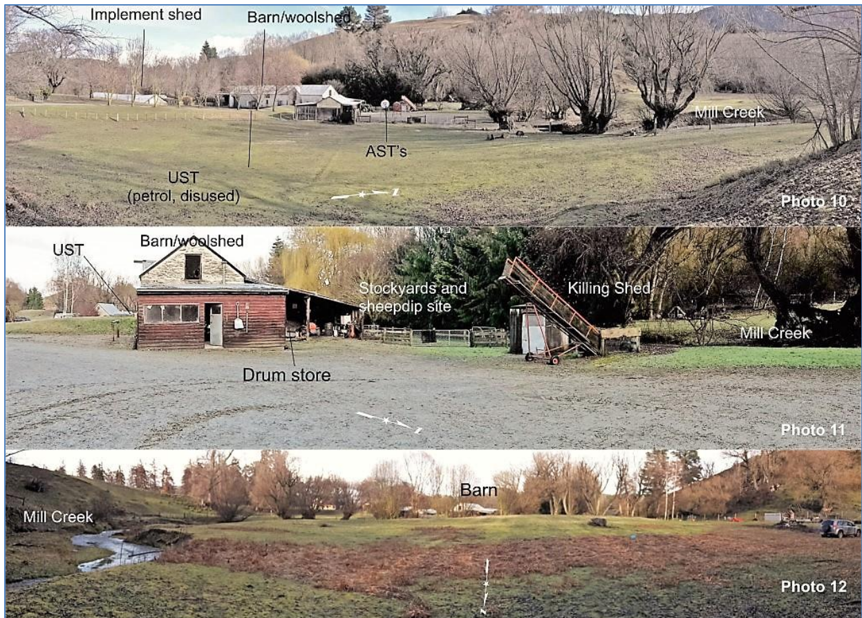
Figure 17; Photos taken from upstream of the farmyard area (immediately proximal to the homestead). Photo 10 shows the farmyard area from the top of the terrace to the east. Photo 11 shows the land to the north of the Barn/woolshed that contains the former sheep dip site, while Photo 12 shows the valley floor upstream of the farmyard. The paddock in Photo 12 has some implements and materials stored in it and the farm manager confirmed that there may be a small farm landfill in a meander at the lower end of this flat immediately upstream from the barn.
