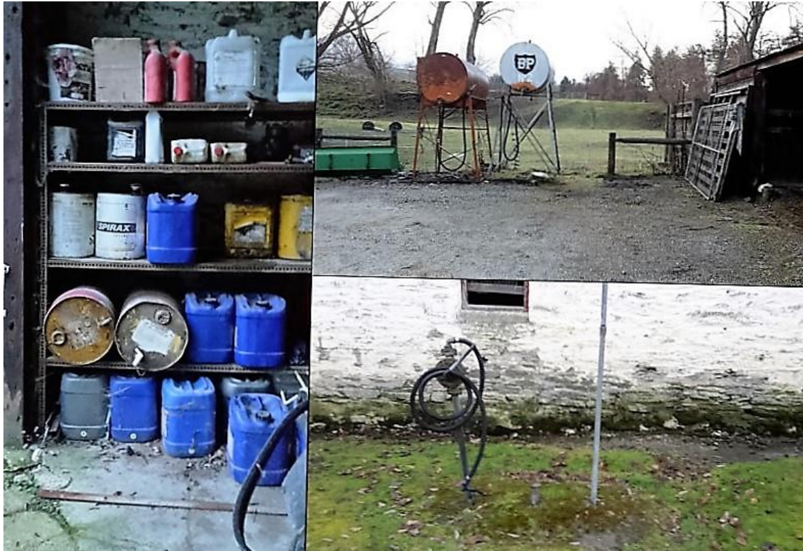
Figure 26: Photos of some of the visual cues for potential contamination that were observed during the site visit; left – drum store adjoining the Barn/woolshed/; top right – the two diesel ASTs by the Shed(stables); and bottom right – evidence of the UST against the eastern wall of the Barn/woolshed.
