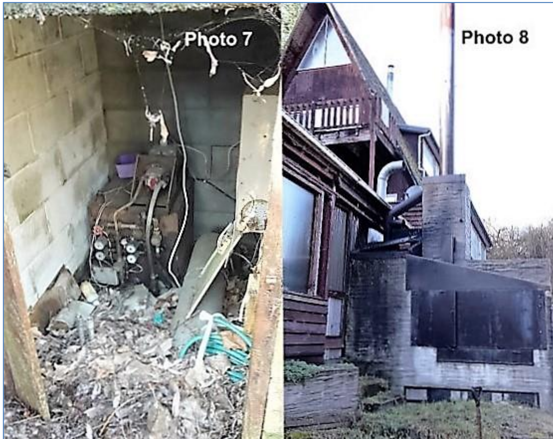
Figure 15: Mill Creek Gorge/Waterfall Park photos with Photo 7 showing the equipment in the shed by the road near the entrance to Waterfall Park, which appears to be some form of fluid pump; Photo 8 shows the A-frame building and the heating furnace.
