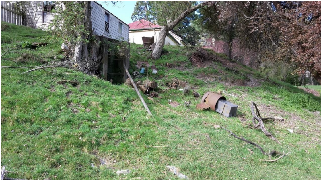
Figure 23: Rubbish on the slope at rear of homestead. Concrete structure and pipe to the left of centre appears to be a septic tank.
