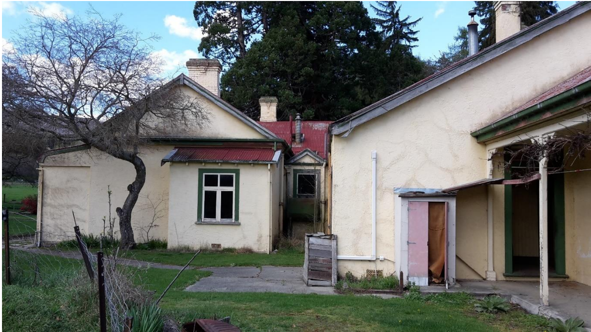
Figure 21: The homestead rear wall and back door with a 500l heating fuel tank on a stand in the recess beside the annex at the centre of the photo.
