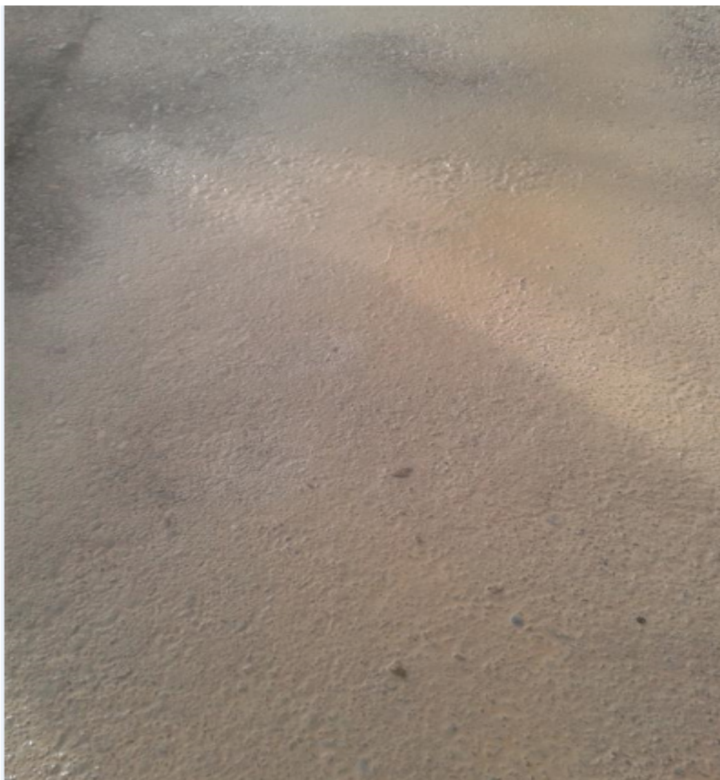
Figure 3 Aggregate wetted down during compaction to achieve 98% of MDD – note no compaction depression lines
