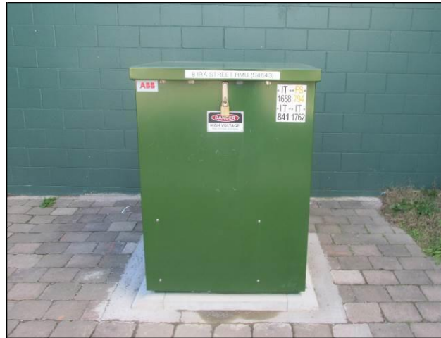
Figure 3: Typical 11kV Ring Main Unit
