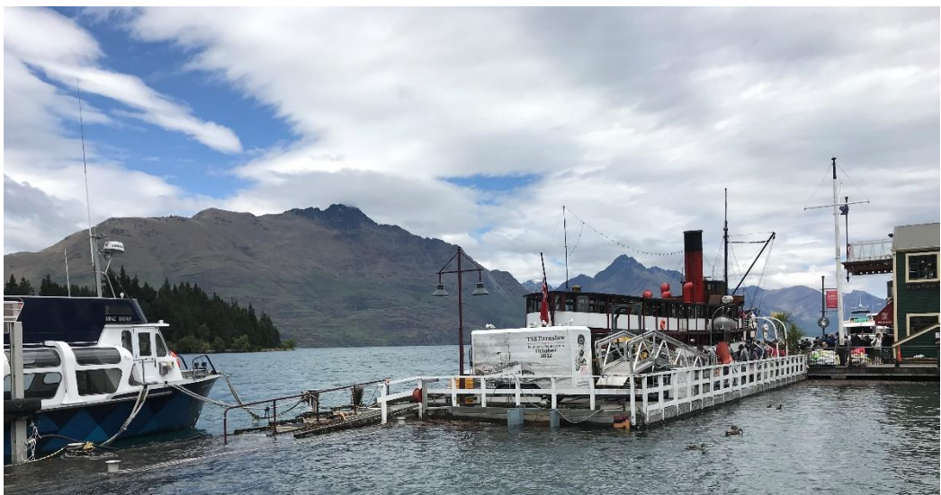
Figure 11 – Photo of Steamer Wharf during December 2019 Flood
