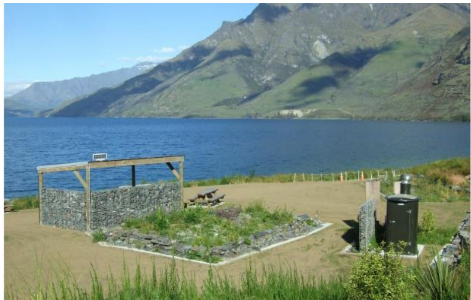
Figure 2 – Photo of Beach Point Picnic Area after completion
